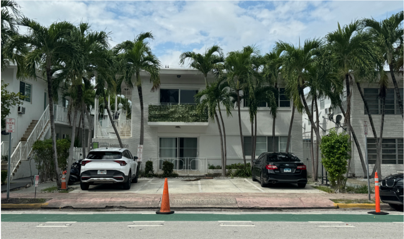
2 1034 PENNSYLVANIA AVE EXISTING ONE-STORY BUILDING
