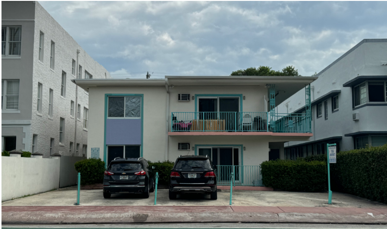
9 1023 PENNSYLVANIA AVE EXISTING TWO-STORY BUILDING
