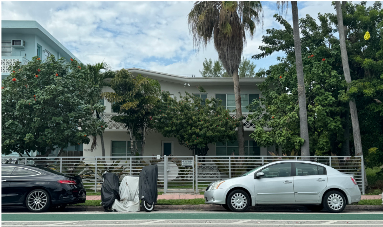
5 1010 PENNSYLVANIA AVE EXISTING TWO-STORY BUILDING
