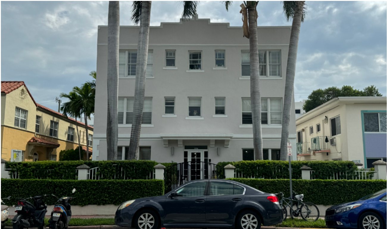
10 1027 PENNSYLVANIA AVE EXISTING THREE-STORY BUILDING
