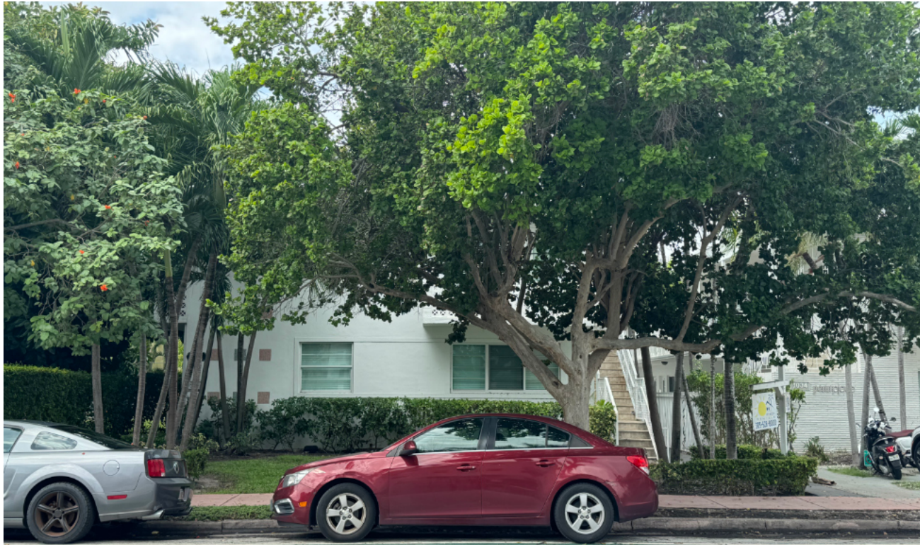
3 1026 PENNSYLVANIA AVE EXISTING TWO-STORY BUILDING
