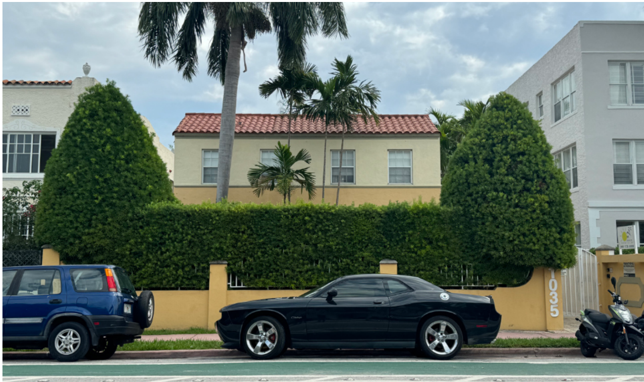
11 1035 PENNSYLVANIA AVE EXISTING TWO-STORY BUILDING
