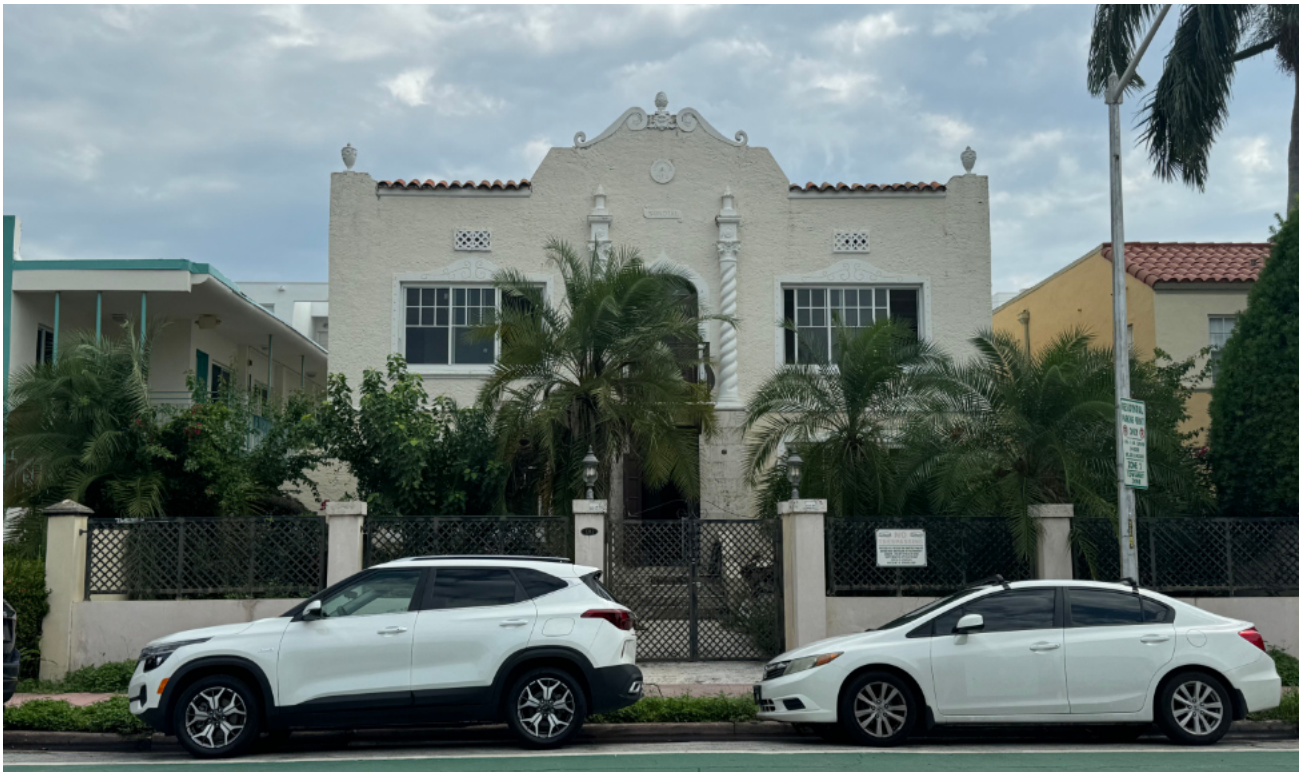
12 1045 PENNSYLVANIA AVE EXISTING TWO-STORY BUILDING
