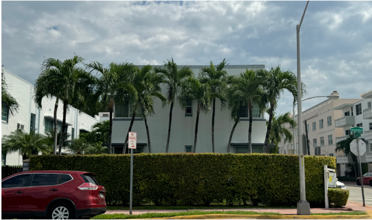
7 1003 PENNSYLVANIA AVE EXISTING TWO-STORY BUILDING
