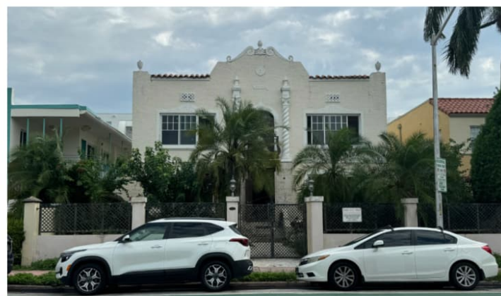
12 1045 PENNSYLVANIA AVE EXISTING TWO-STORY BUILDING
