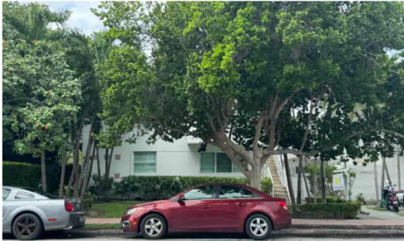
3 1026 PENNSYLVANIA AVE EXISTING TWO-STORY BUILDING
