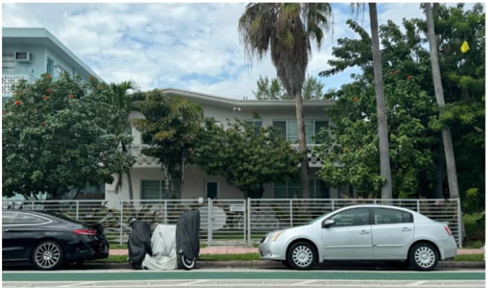
5 1010 PENNSYLVANIA AVE EXISTING TWO-STORY BUILDING
