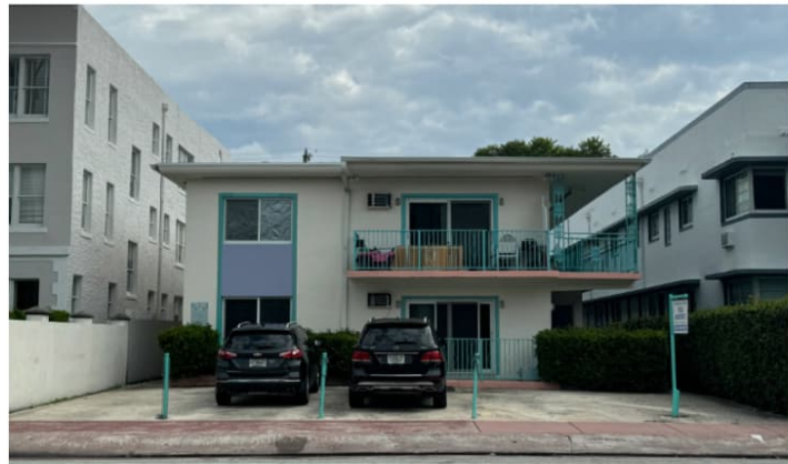
9 1023 PENNSYLVANIA AVE EXISTING TWO-STORY BUILDING
