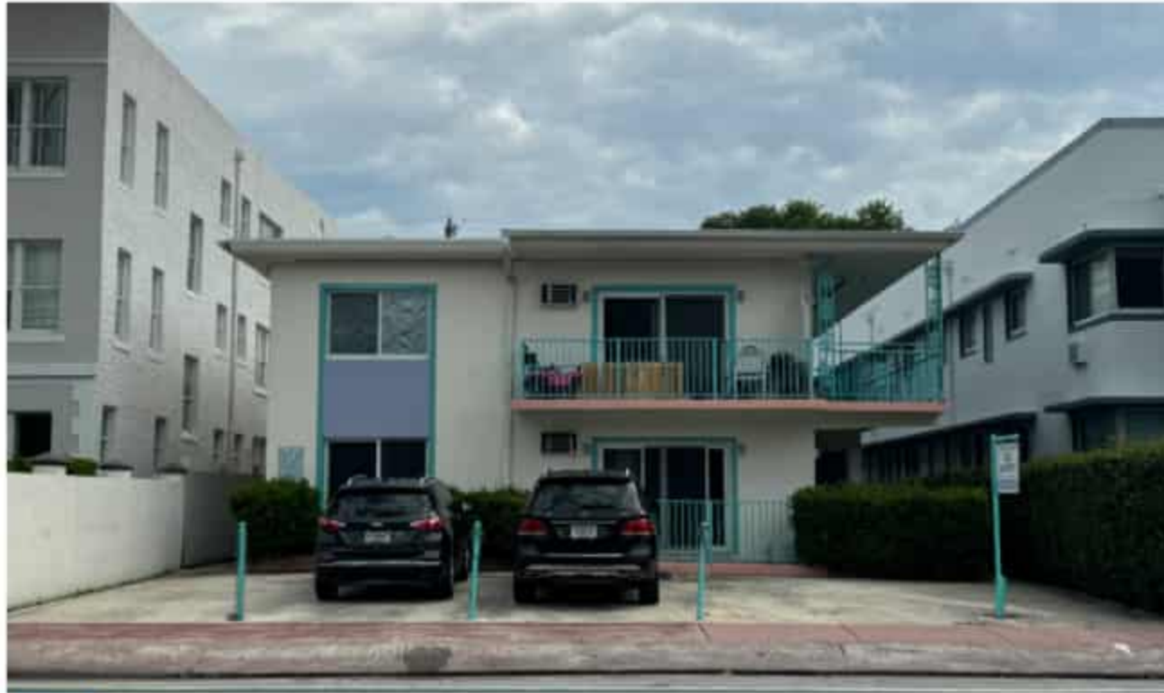
9 1023 PENNSYLVANIA AVE EXISTING TWO-STORY BUILDING
