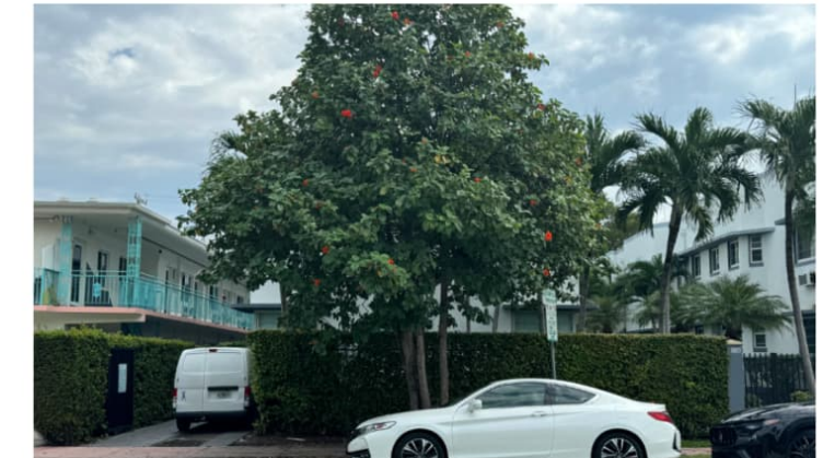
8 1005 PENNSYLVANIA AVE EXISTING TWO-STORY BUILDING
