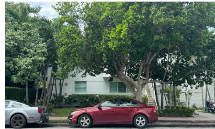
3 1026 PENNSYLVANIA AVE EXISTING TWO-STORY BUILDING
