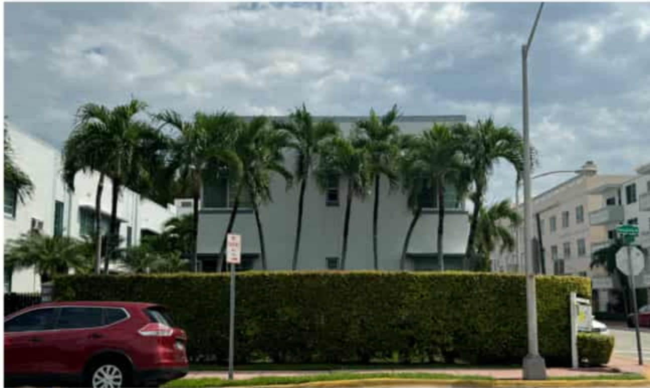
7 1003 PENNSYLVANIA AVE EXISTING TWO-STORY BUILDING
