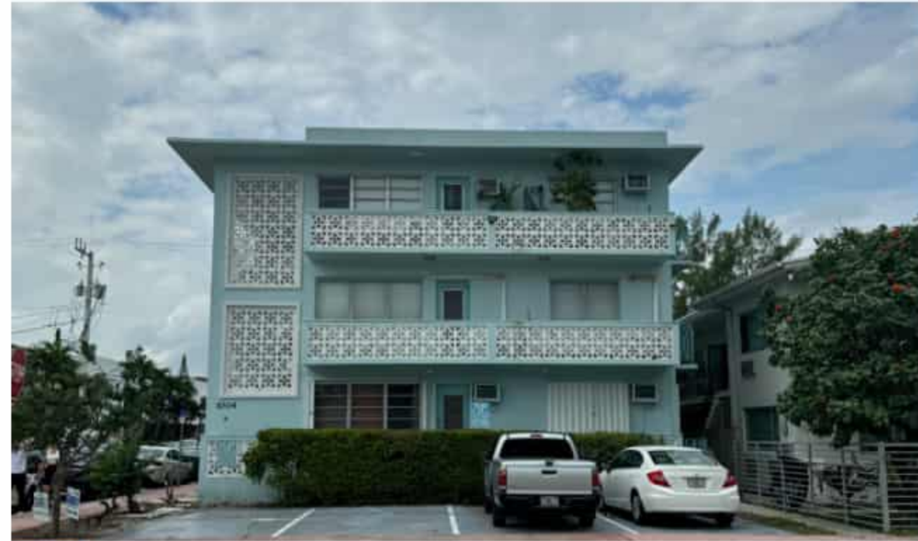
6 1004 PENNSYLVANIA AVE EXISTING THREE-STORY BUILDING
