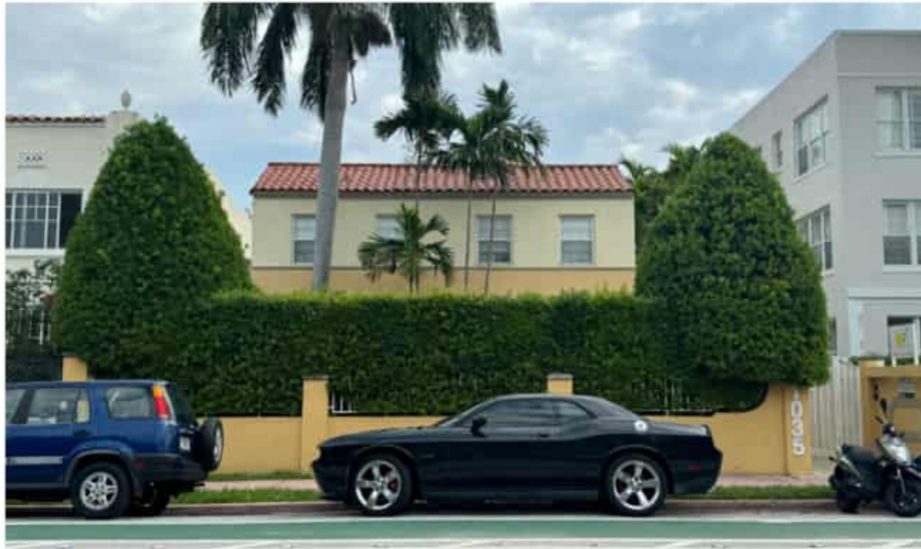
11 1035 PENNSYLVANIA AVE EXISTING TWO-STORY BUILDING
