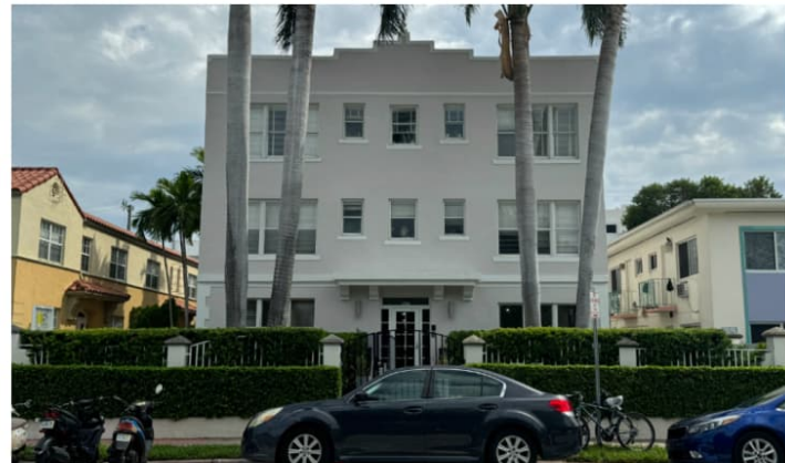
10 1027 PENNSYLVANIA AVE EXISTING THREE-STORY BUILDING
