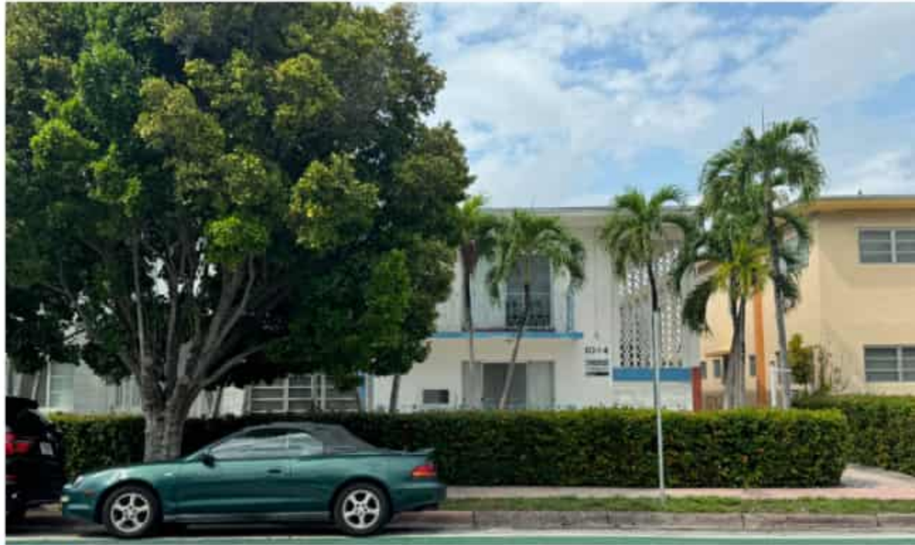
1 1044 PENNSYLVANIA AVE EXISTING TWO-STORY BUILDING
