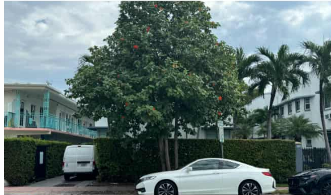
8 1005 PENNSYLVANIA AVE EXISTING TWO-STORY BUILDING
