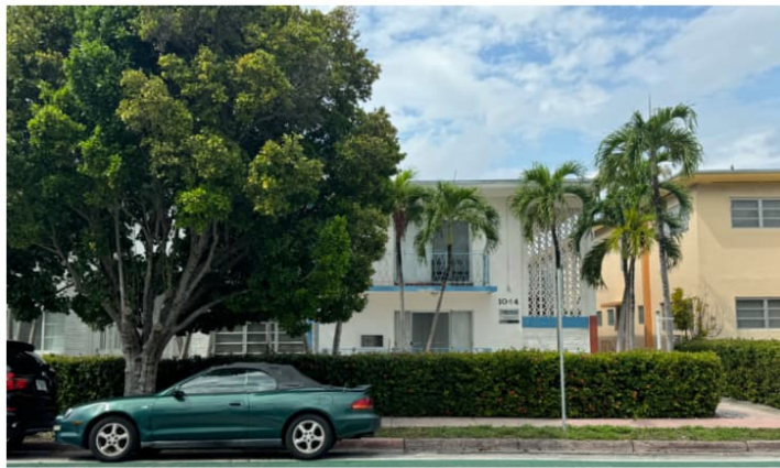
1 1044 PENNSYLVANIA AVE EXISTING TWO-STORY BUILDING
