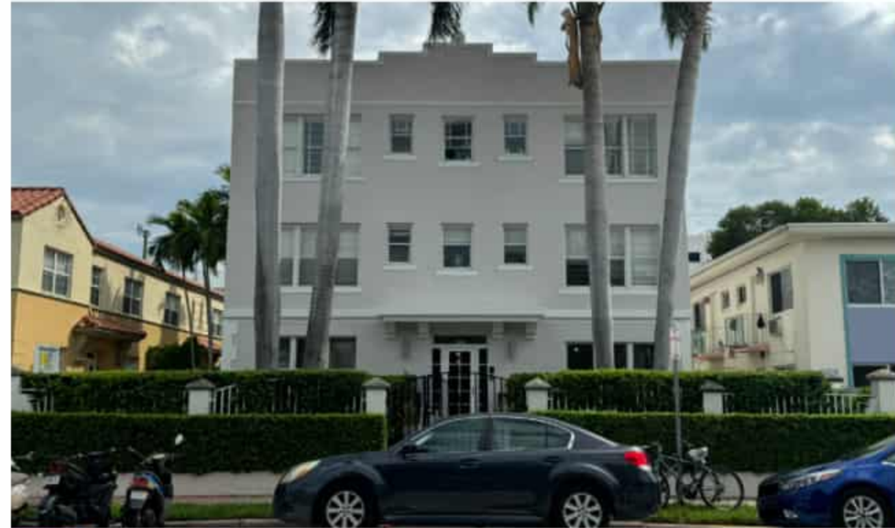
10 1027 PENNSYLVANIA AVE EXISTING THREE-STORY BUILDING
