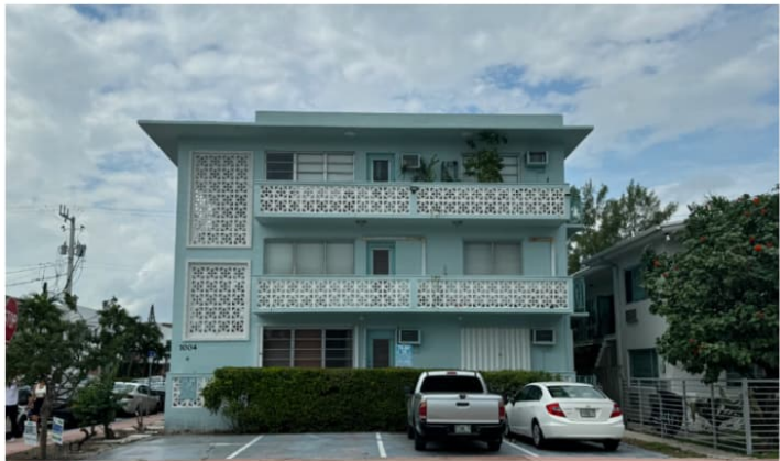
6 1004 PENNSYLVANIA AVE EXISTING THREE-STORY BUILDING
