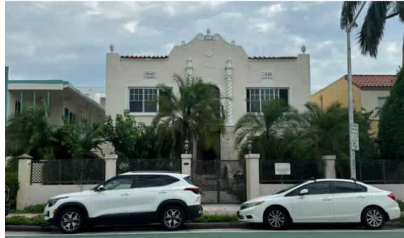
12 1045 PENNSYLVANIA AVE EXISTING TWO-STORY BUILDING
