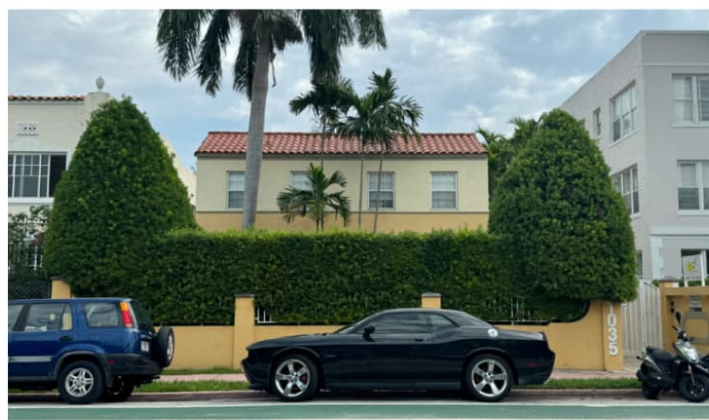
11 1035 PENNSYLVANIA AVE EXISTING TWO-STORY BUILDING
