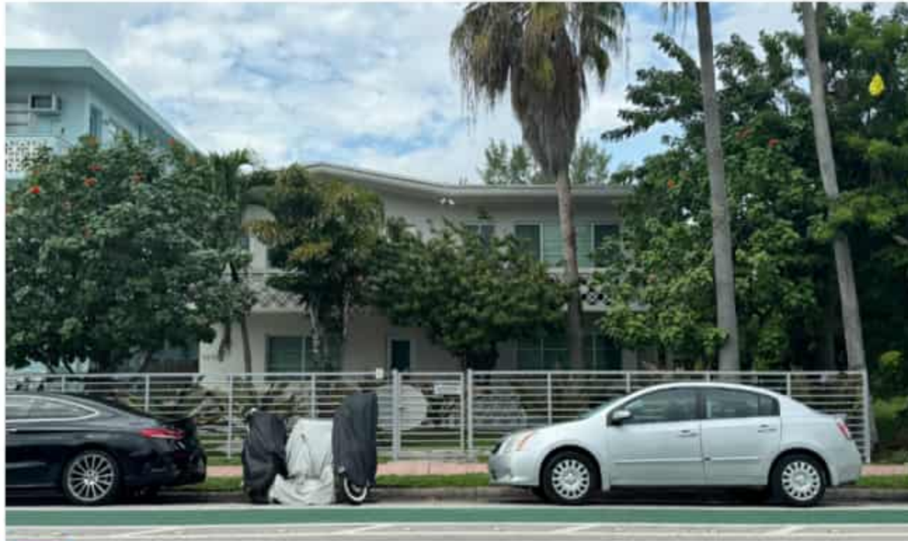
5 1010 PENNSYLVANIA AVE EXISTING TWO-STORY BUILDING
