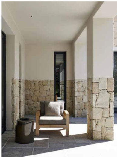
WHITE STUCCO, CORAL ROCK REVEALS AND DETAIL
