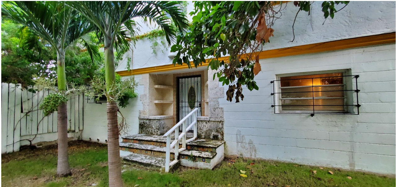
VIEW OF EXISTING MAIN ENTRY
