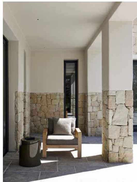
WHJITE STUCCO, CORAL ROCK REVEALS AND DETAIL
