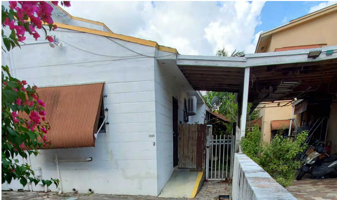
9 VIEW OF LOT 1800 FACING WEST 1 1/2" = 1'-0"
