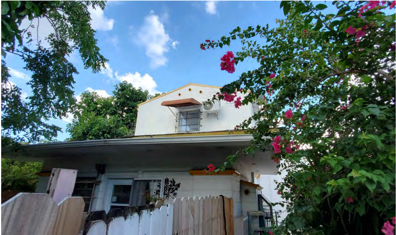
1 VIEW OF LOT 1800 FACING WEST 1 1/2" = 1'-0"
