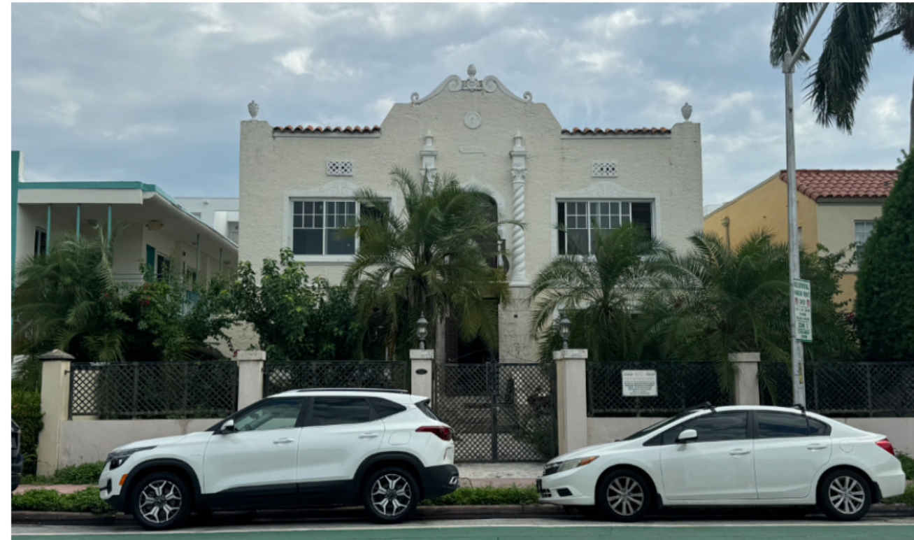
12 1045 PENNSYLVANIA AVE EXISTING TWO-STORY BUILDING
