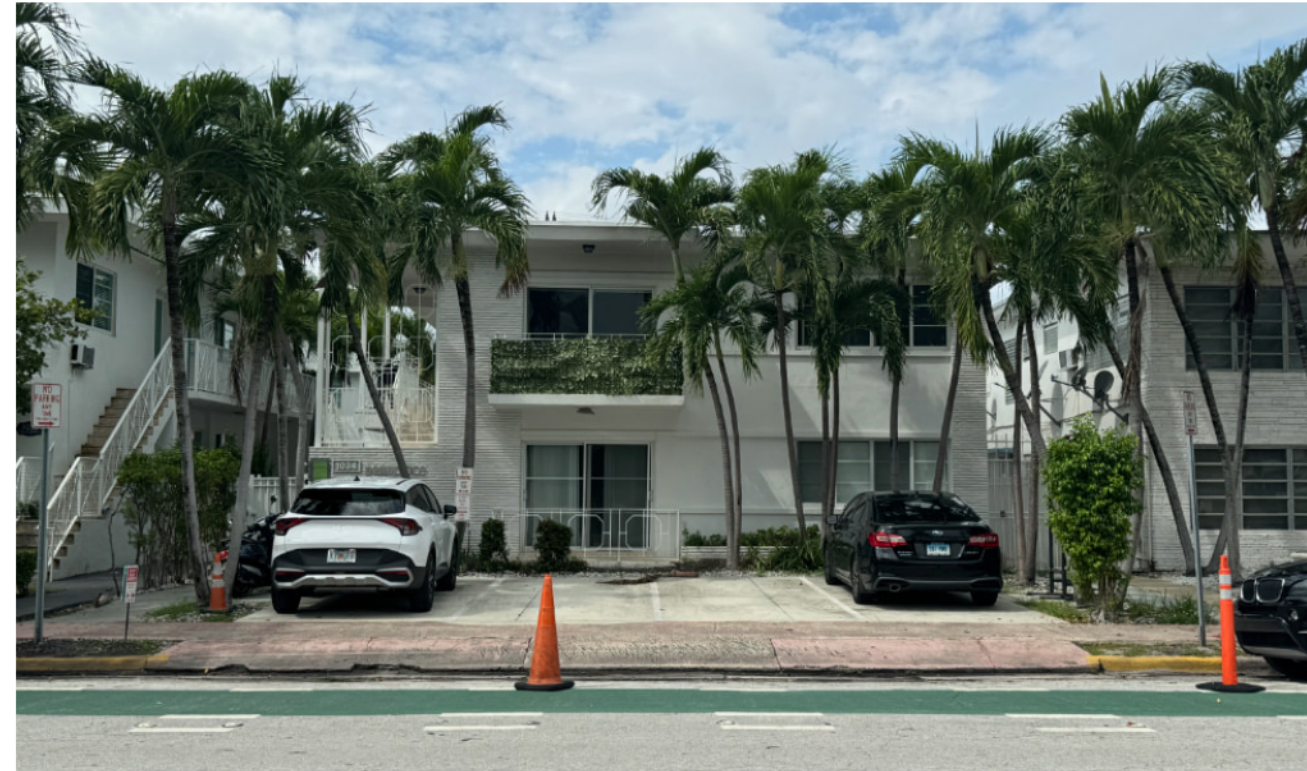
2 1034 PENNSYLVANIA AVE EXISTING ONE-STORY BUILDING
