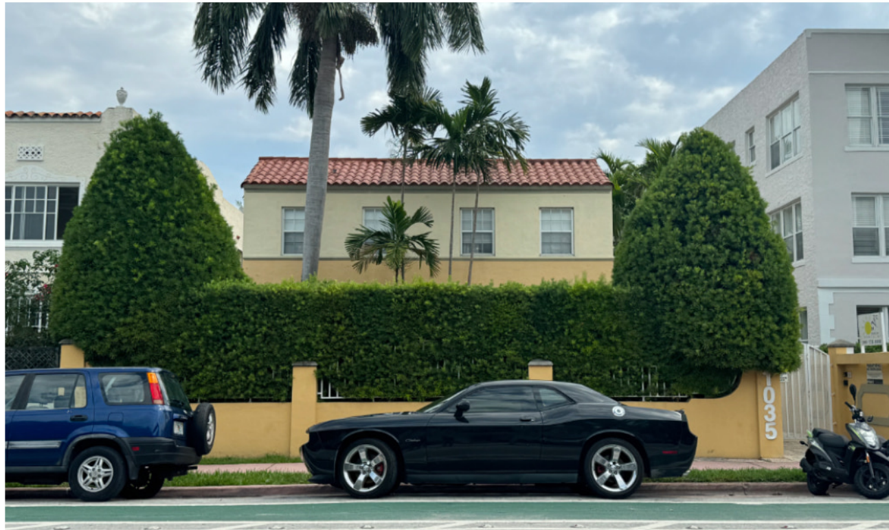
11 1035 PENNSYLVANIA AVE EXISTING TWO-STORY BUILDING
