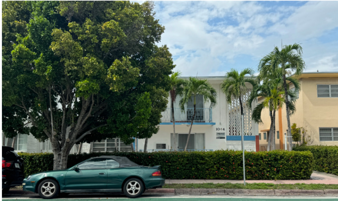
1 1044 PENNSYLVANIA AVE EXISTING TWO-STORY BUILDING
