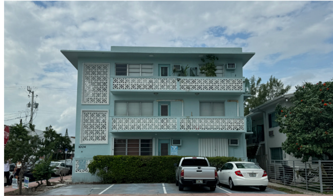
6 1004 PENNSYLVANIA AVE EXISTING THREE-STORY BUILDING
