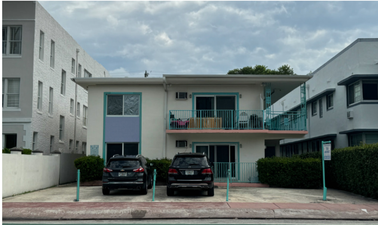
9 1023 PENNSYLVANIA AVE EXISTING TWO-STORY BUILDING
