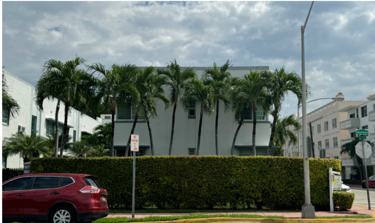
7 1003 PENNSYLVANIA AVE EXISTING TWO-STORY BUILDING
