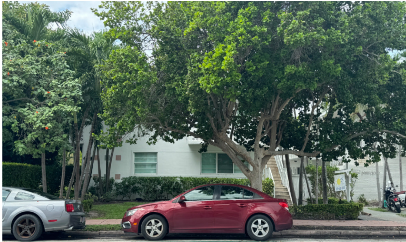
3 1026 PENNSYLVANIA AVE EXISTING TWO-STORY BUILDING
