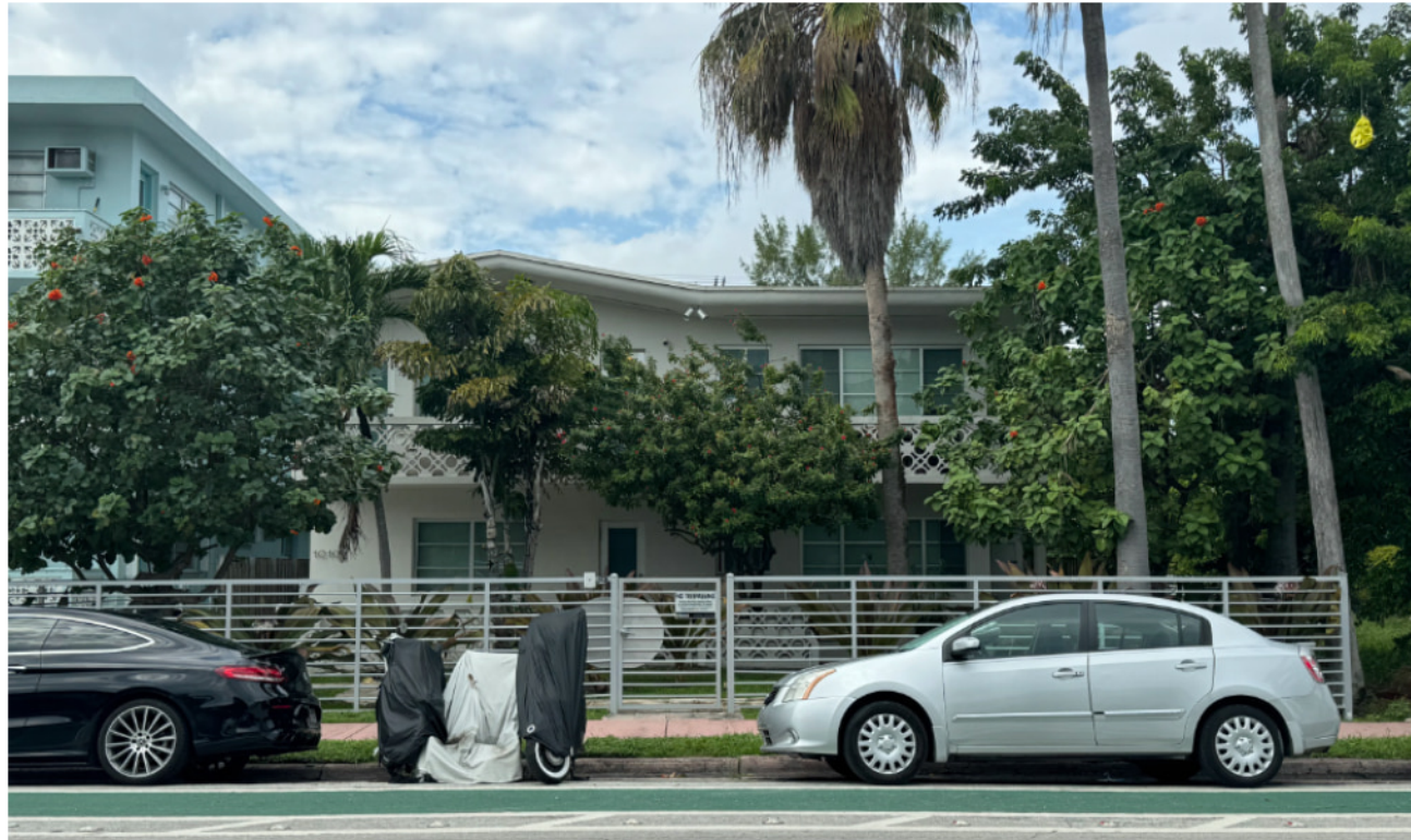
5 1010 PENNSYLVANIA AVE EXISTING TWO-STORY BUILDING
