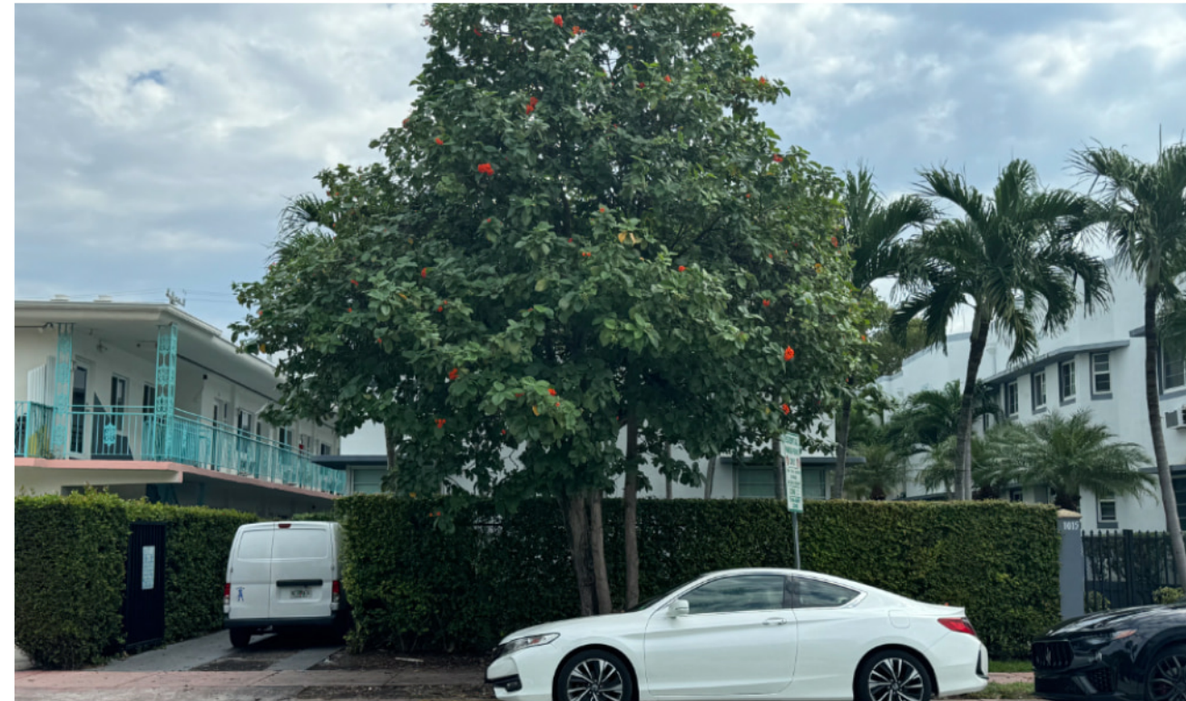
8 1005 PENNSYLVANIA AVE EXISTING TWO-STORY BUILDING
