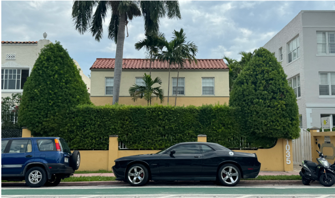
11 1035 PENNSYLVANIA AVE EXISTING TWO-STORY BUILDING
