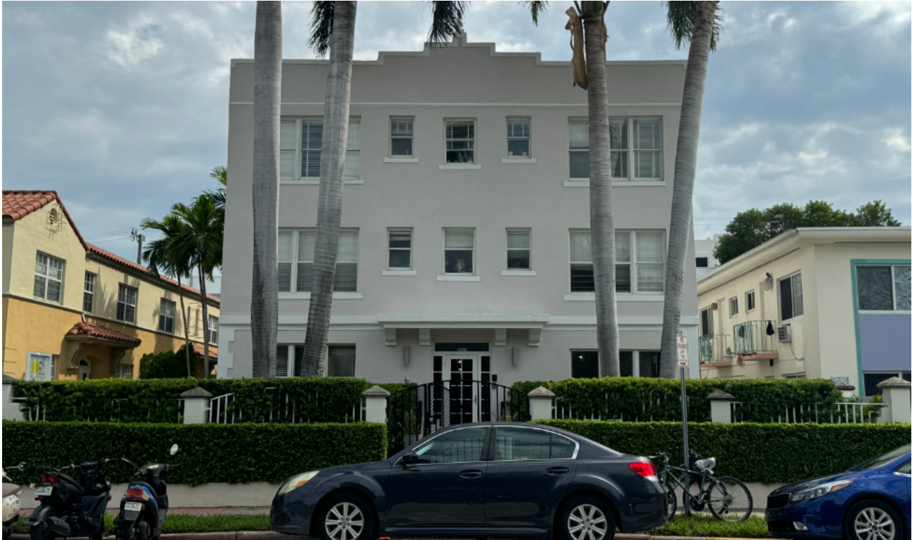
10 1027 PENNSYLVANIA AVE EXISTING THREE-STORY BUILDING
