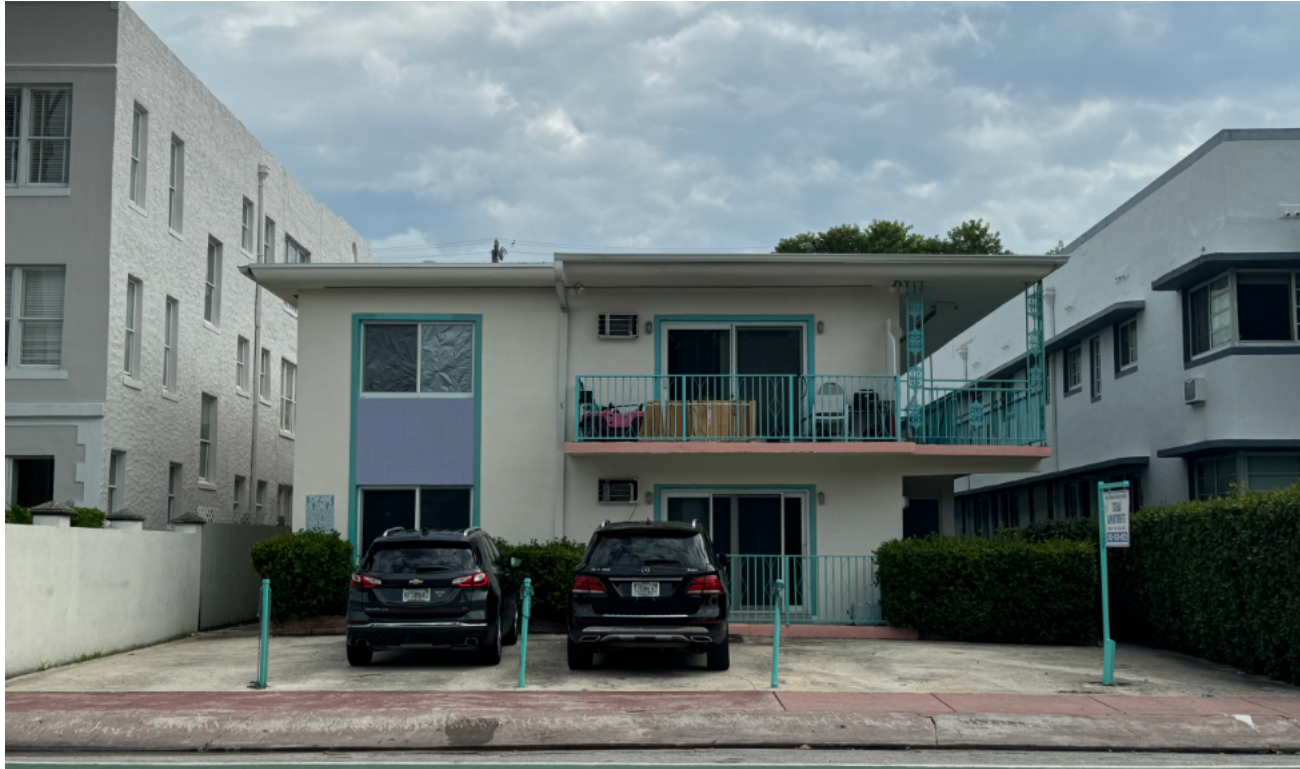
9 1023 PENNSYLVANIA AVE EXISTING TWO-STORY BUILDING
