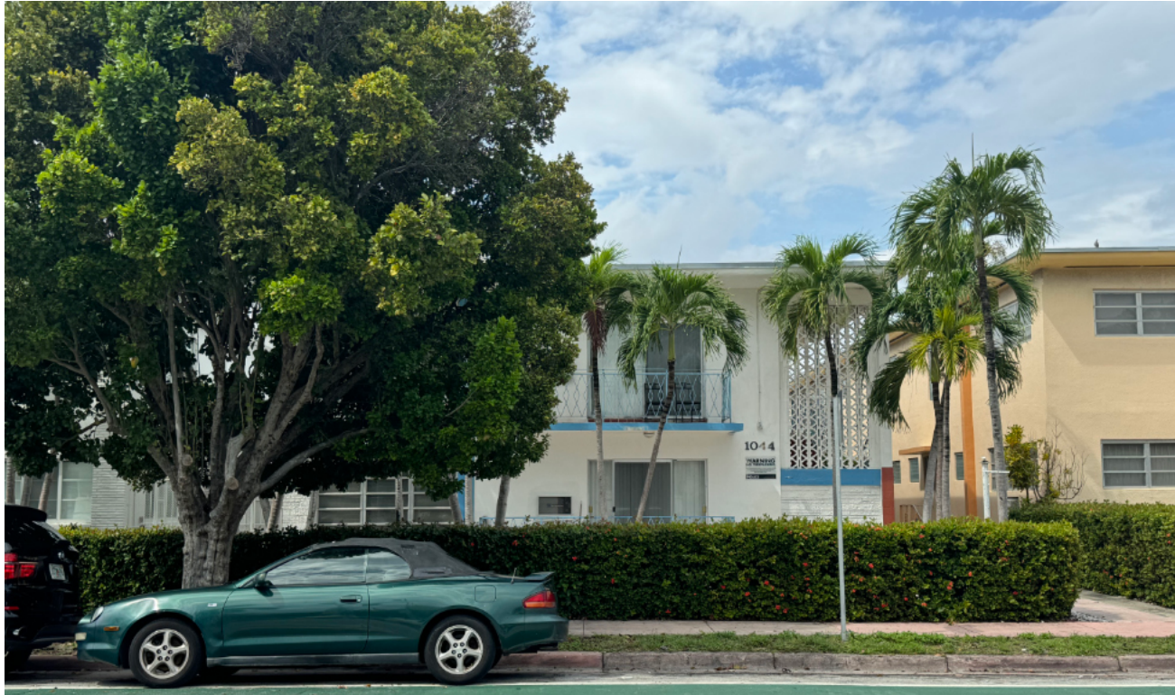
1 1044 PENNSYLVANIA AVE EXISTING TWO-STORY BUILDING
