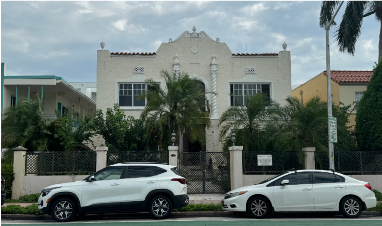
12 1045 PENNSYLVANIA AVE EXISTING TWO-STORY BUILDING
