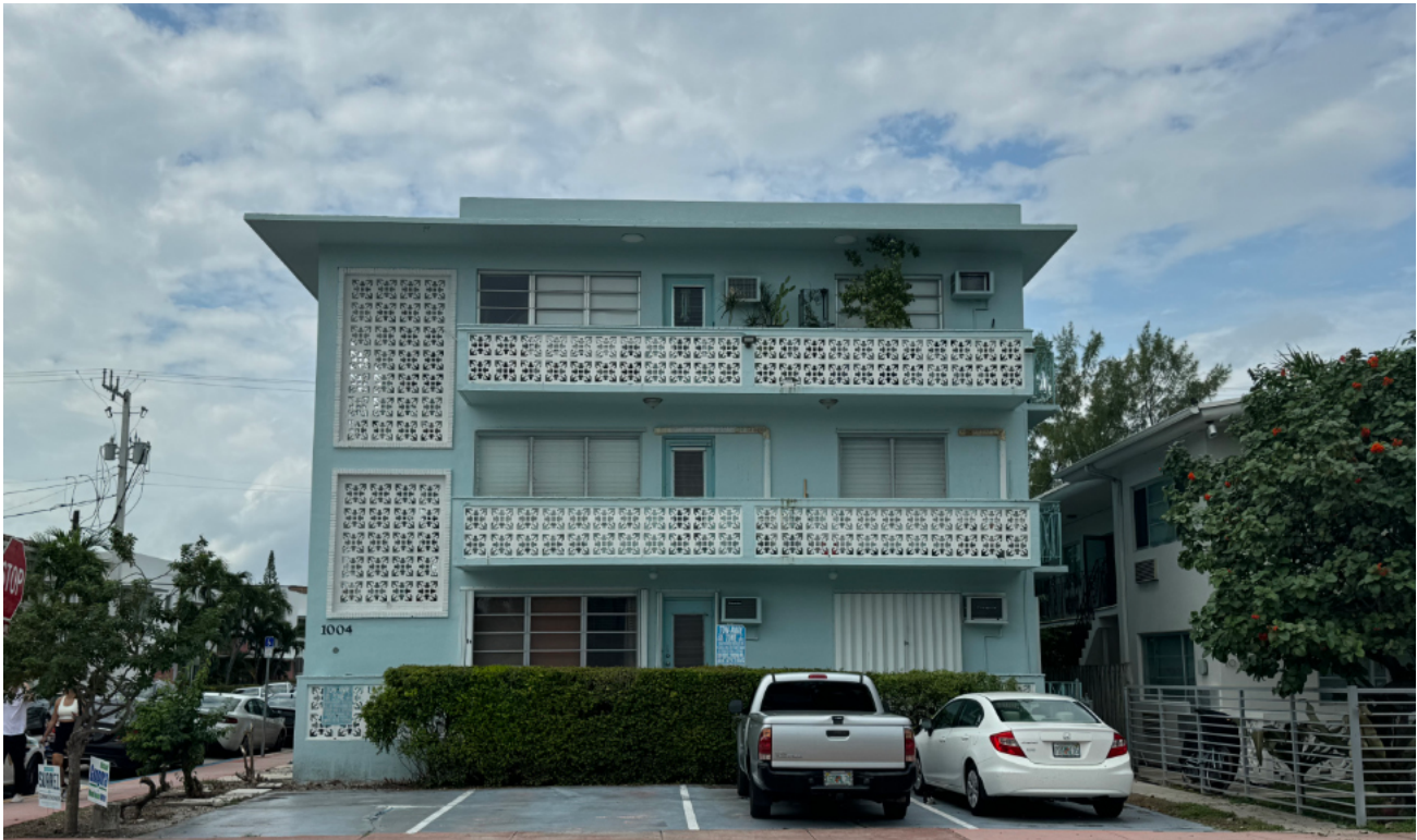
6 1004 PENNSYLVANIA AVE EXISTING THREE-STORY BUILDING
