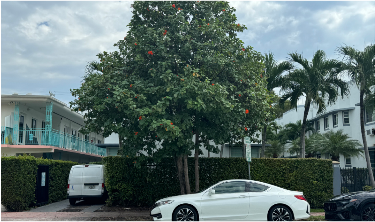
8 1005 PENNSYLVANIA AVE EXISTING TWO-STORY BUILDING
