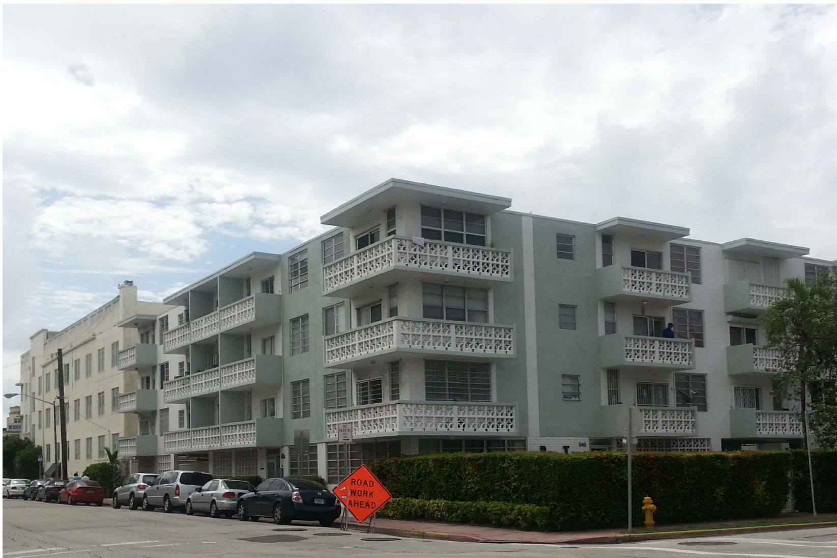
4 SE CORNER BUILDING PENNSYLVANIA AVE & 10 ST
