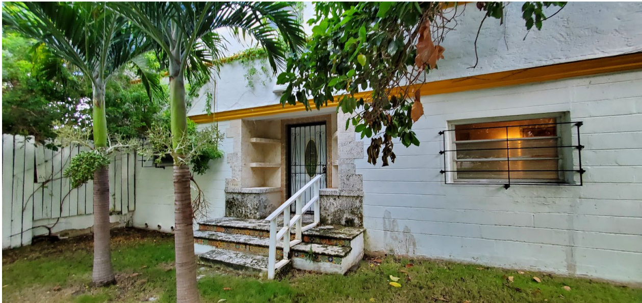
VIEW OF EXISTING MAIN ENTRY
