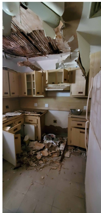
3 INTERIOR OF HOUSE 2 1" = 20'-0"
