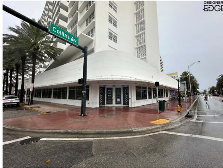
CORNER OF COLLINS AVENUE AND LINCOLN ROAD
