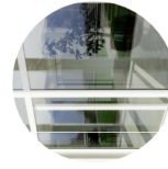
2 | ALUMINUM FRAME WHITE OPULENCE OC-89 BENJAMIN MOORE / OR EQUIVALENT APPROVED BY ARCHITECT
