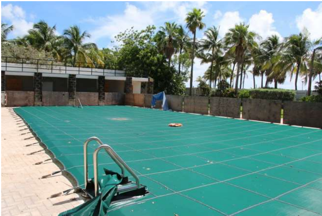
PHOTO BELOW: POOL AREA WITH PARTIALLY RE-CONSTRUCTED CABANAS AT REAR LEFT. (22)
