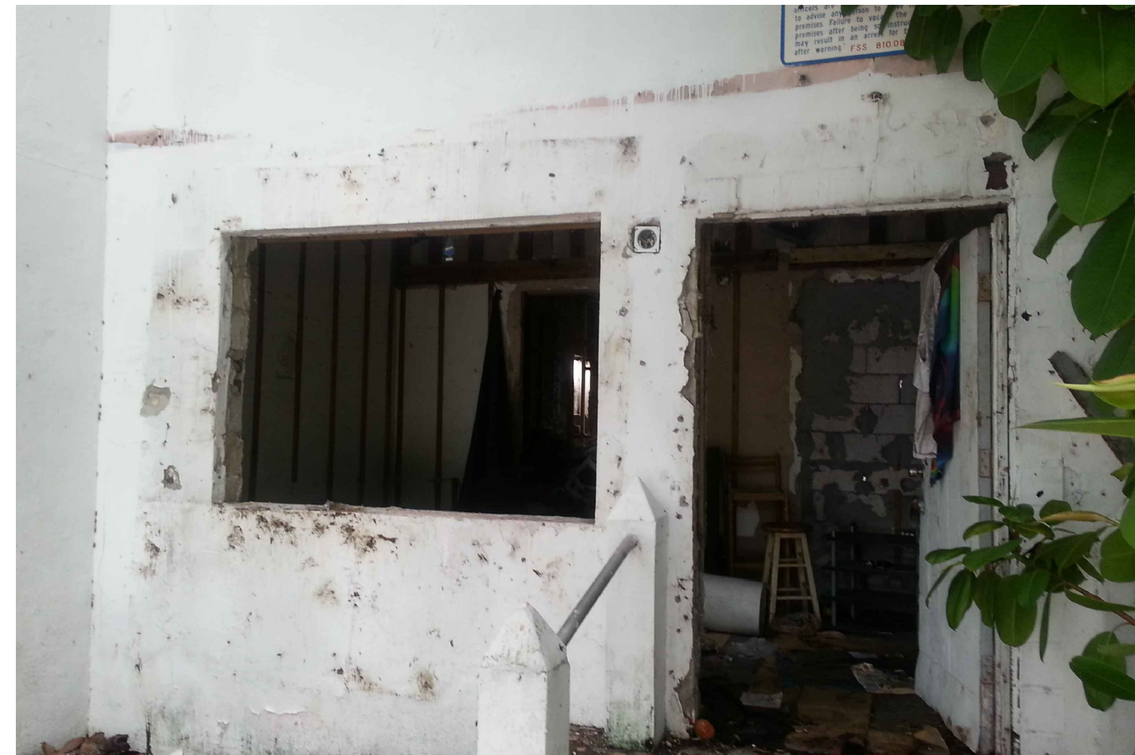
5 EAST BUILDING WEST ENTRANCE
