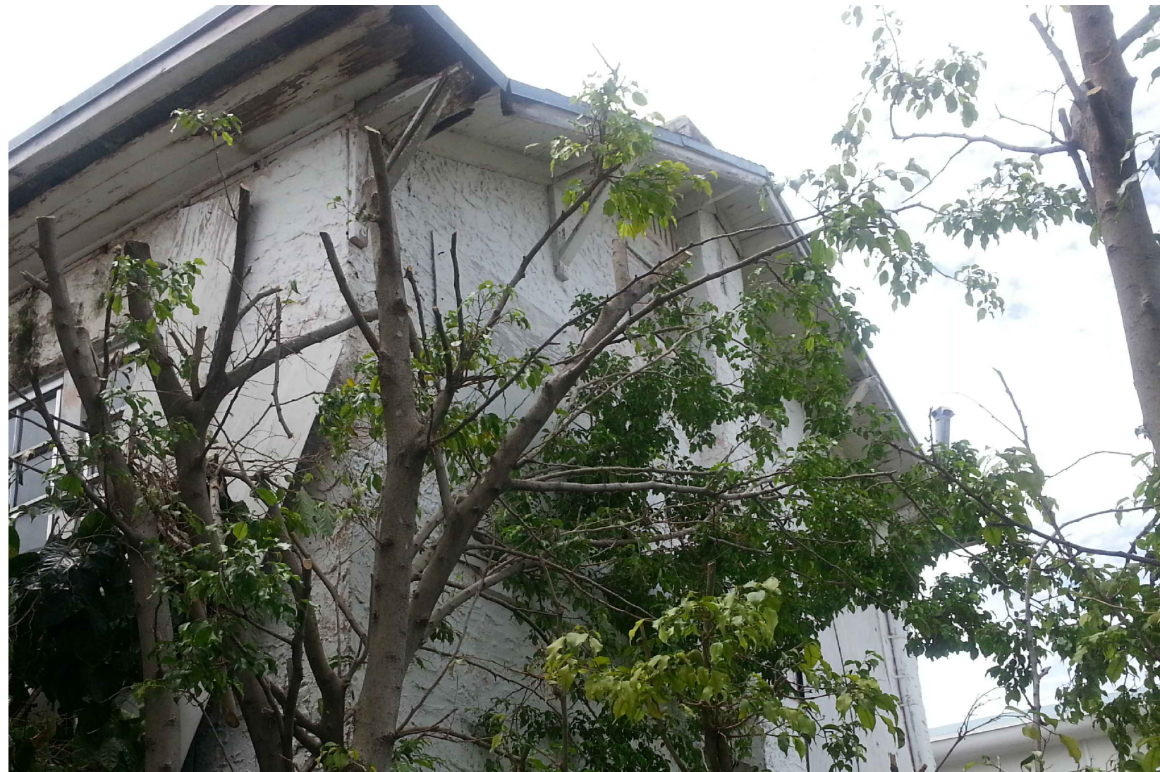
4 EAST BUILDING NW CONER VIEW
