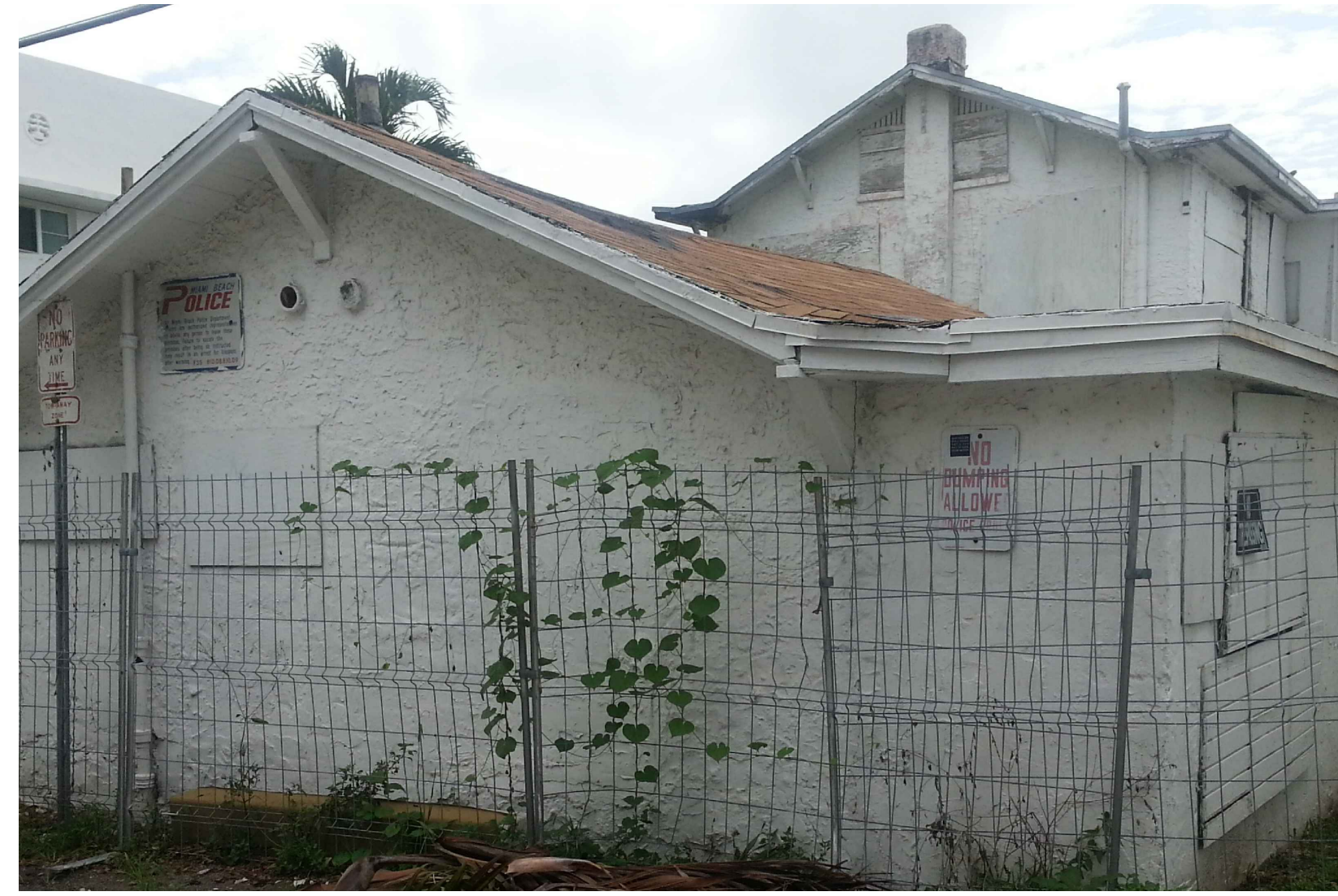
2 BUILDING VIEW FROM SW CORNER
