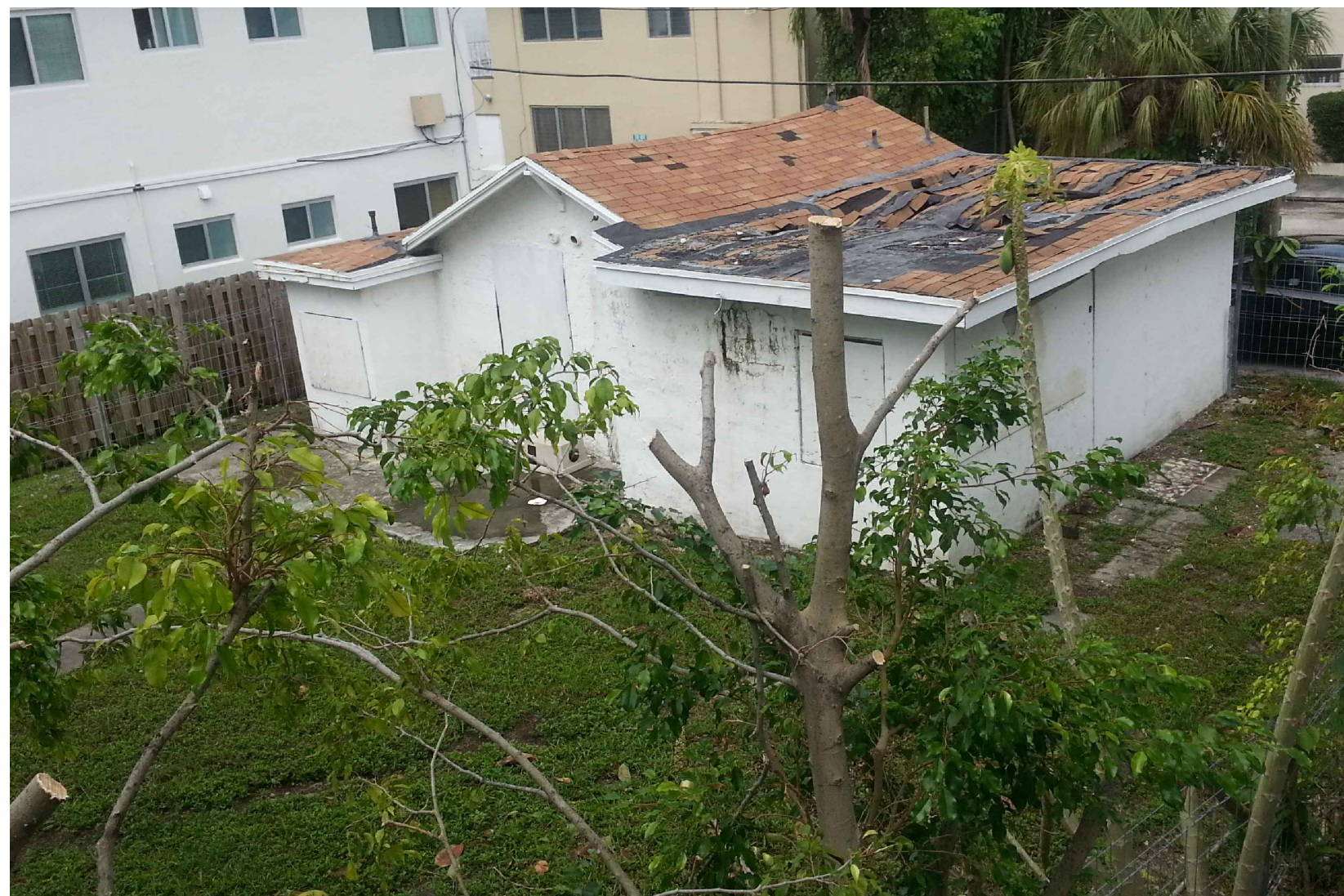
7 WEST BUILDING FROM NE CORNER
