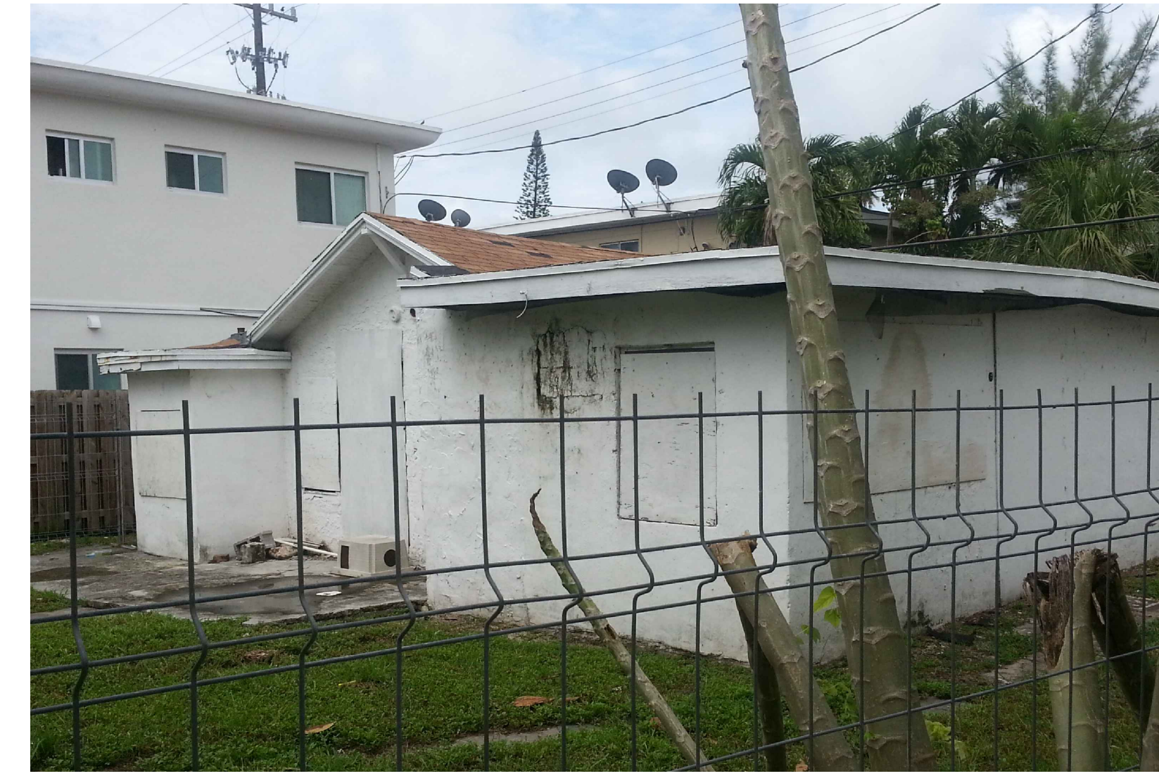
3 BUILDING VIEW FROM NW CORNER
