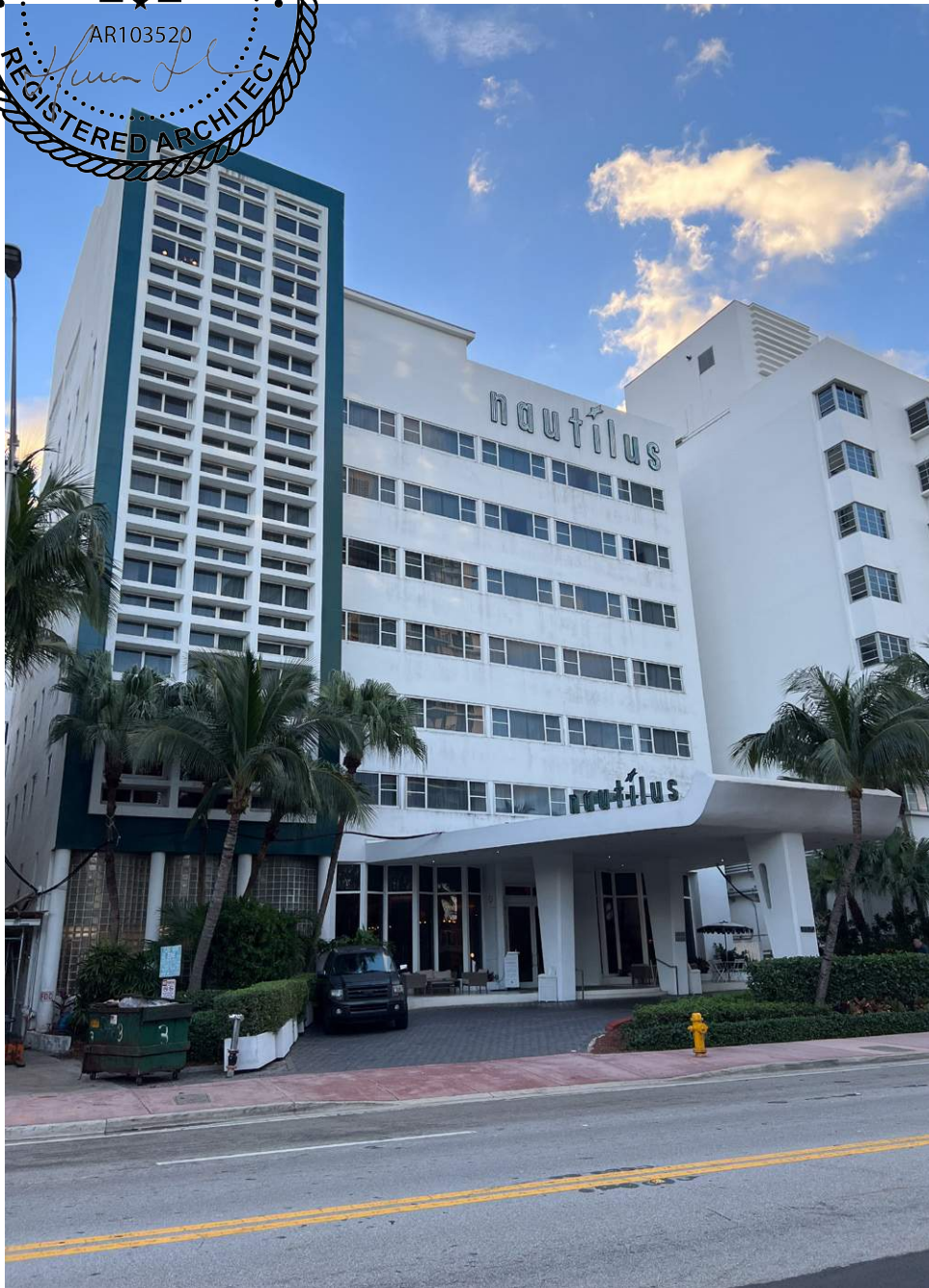
01 EXTERIOR - ENTRANCE (WEST) FACADE - 01.03.24
