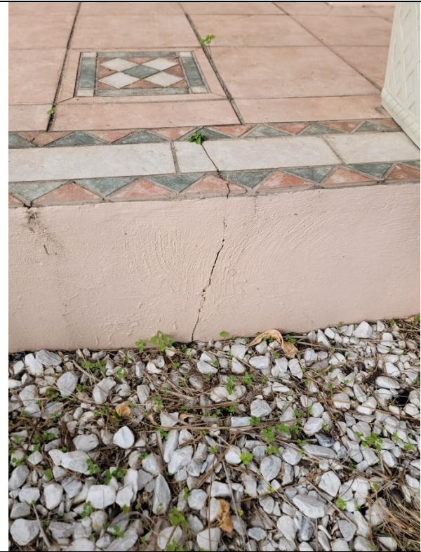
Foundation cracking
