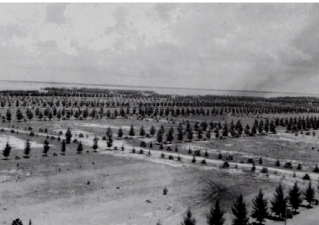
TOP PHOTO: 1905 CLEARING THE FUTURE LINCOLN ROAD (8)
