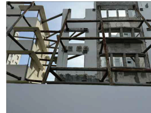
PHOTO #1-EXTERIOR SHORING N.T.S.
