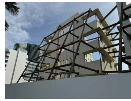
PHOTO #2- EXTERIOR SHORING N.T.S
