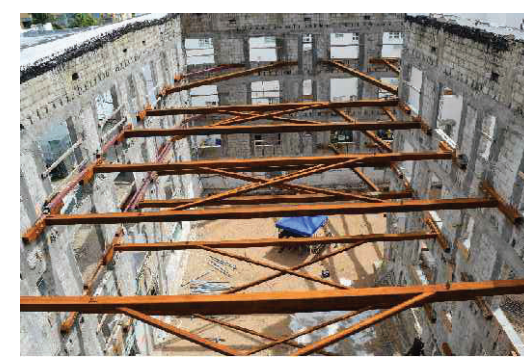
PHOTO #3- INTERIOR SHORING N.T.S
