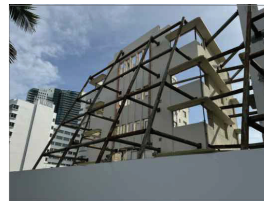
PHOTO #2- EXTERIOR SHORING N.T.S.
