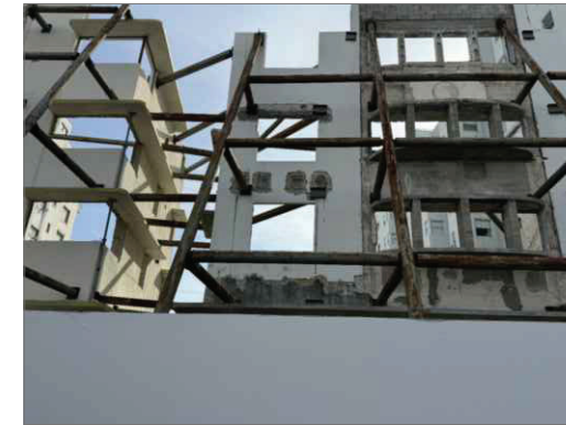
PHOTO #1-EXTERIOR SHORING N.T.S
