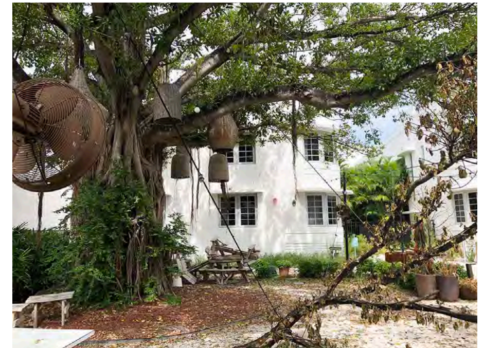
Banyan Tree relative to the Campton Apts West Facade.
