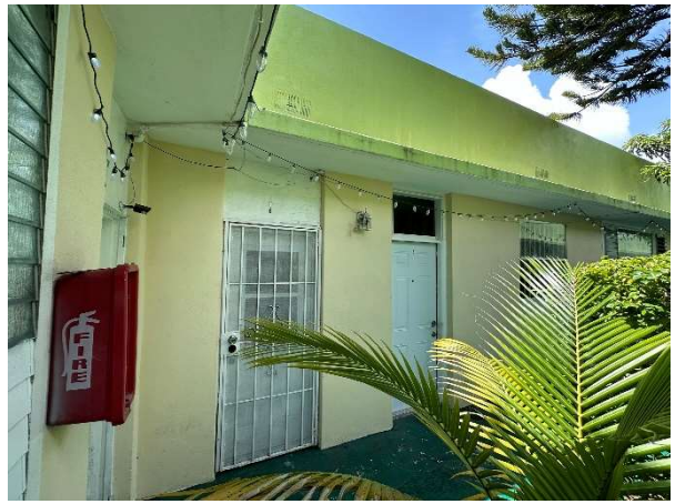
Figure 98. View of Unit 6, looking southeast, August 2023.
