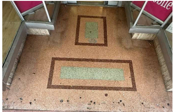
Figure 61. Detail of terrazzo floor at entrance to 1507 Washington Avenue, August 2023.
