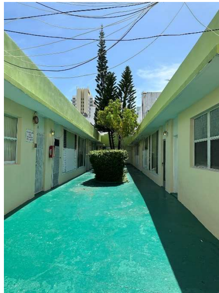
Figure 92. View of courtyard at interior of “U” at rear building, looking east, August 2023.
