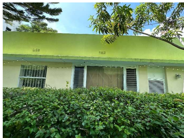
Figure 96. View of Unit 4, looking south, August 2023.
