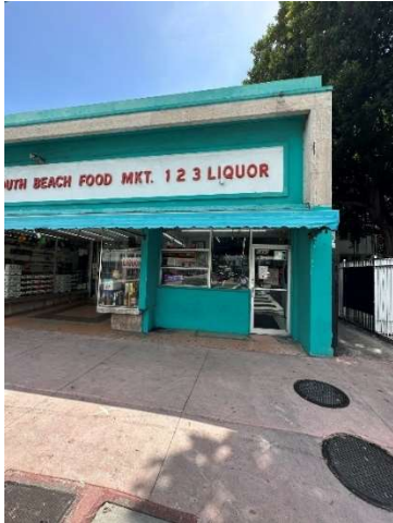
Figure 41. View of 1491 Washington Avenue, August 2023.
