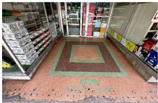
Figure 53. Detail of terrazzo floor at entrance to 1493 Washington Avenue, August 2023.
