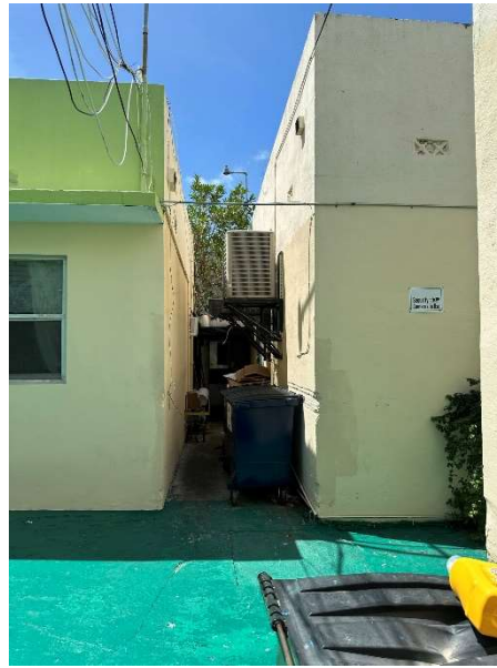
Figure 90. View of narrow walkway between south front building and rear building, looking south, August 2023.
