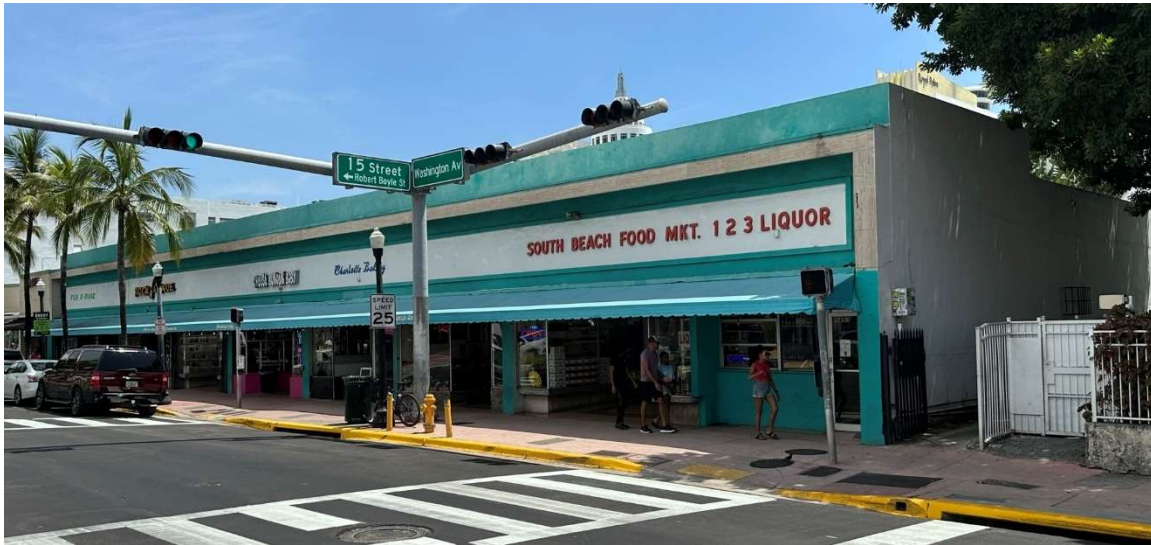
Figure 38. View of 1491-1513 Washington Avenue, looking northeast, August 2023.
