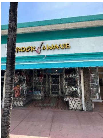
Figure 47. View of 1509 Washington Avenue, August 2023.
