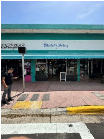
Figure 44. View of 1499 Washington Avenue, August 2023.
