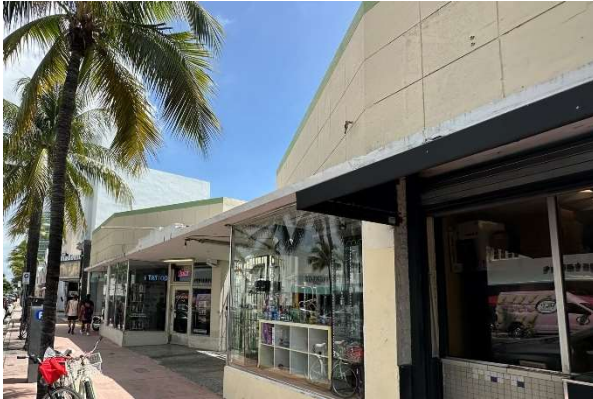
Figure 72. Detail of continuous concrete canopy, August 2023.
