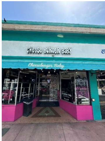
Figure 45. View of 1505 Washington Avenue, August 2023.
