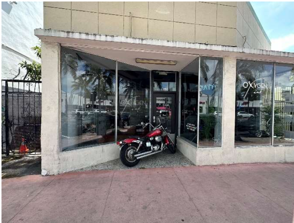
Figure 83. View of 1523 Washington Avenue, looking east, August 2023.
