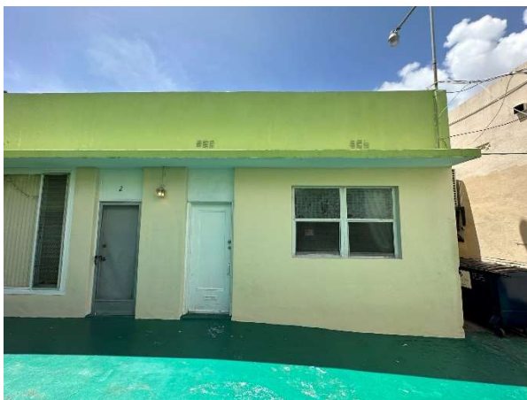
Figure 93. View of Unit 1, looking south, August 2023.
