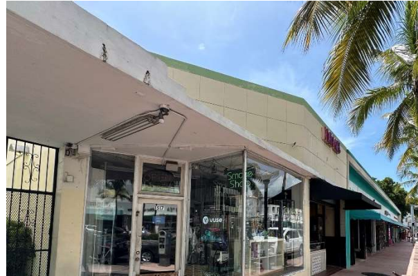
Figure 73. Detail of storefront extension under continuous canopy, August 2023.
