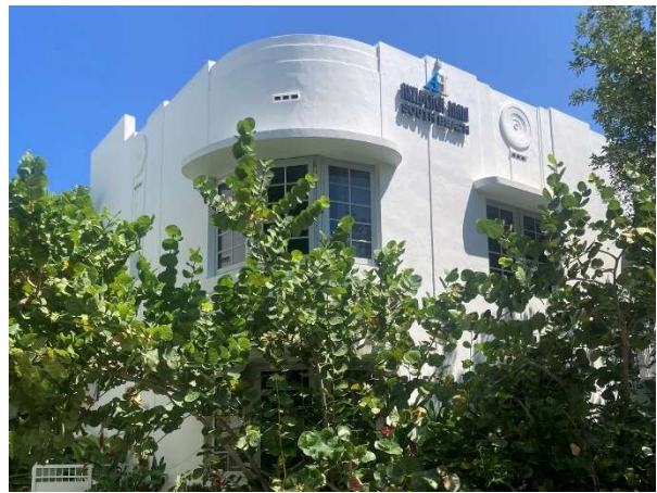
Figure 38. Detail of rounded corner and eyebrow, September 2023.
