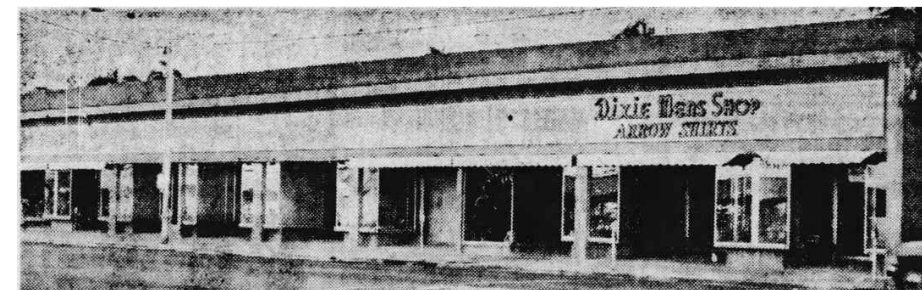
AT MIAMI BEACH, this new commercial building, containing nine store units, has just been completed at 15th st. and Washington ave. for Daniel I. Taradash. Constructed by the Leifer Construction Co. from plans drawn by Architect Albert Anis, the building front 140 feet on Washington ave. and extends 80 feet in depth. Management of the building is by Taradash Properties, 927 Lincoln rd.
