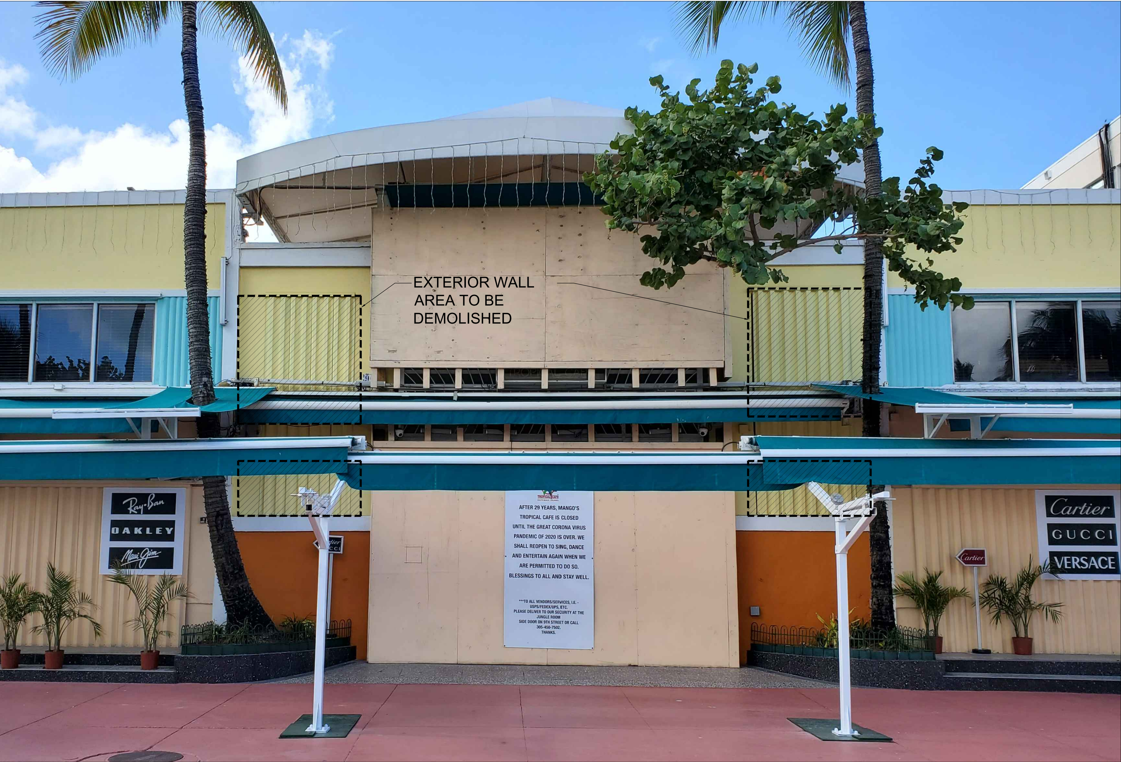
A1 EXTERIOR WALL AREA TO BE DEMOLISHED
