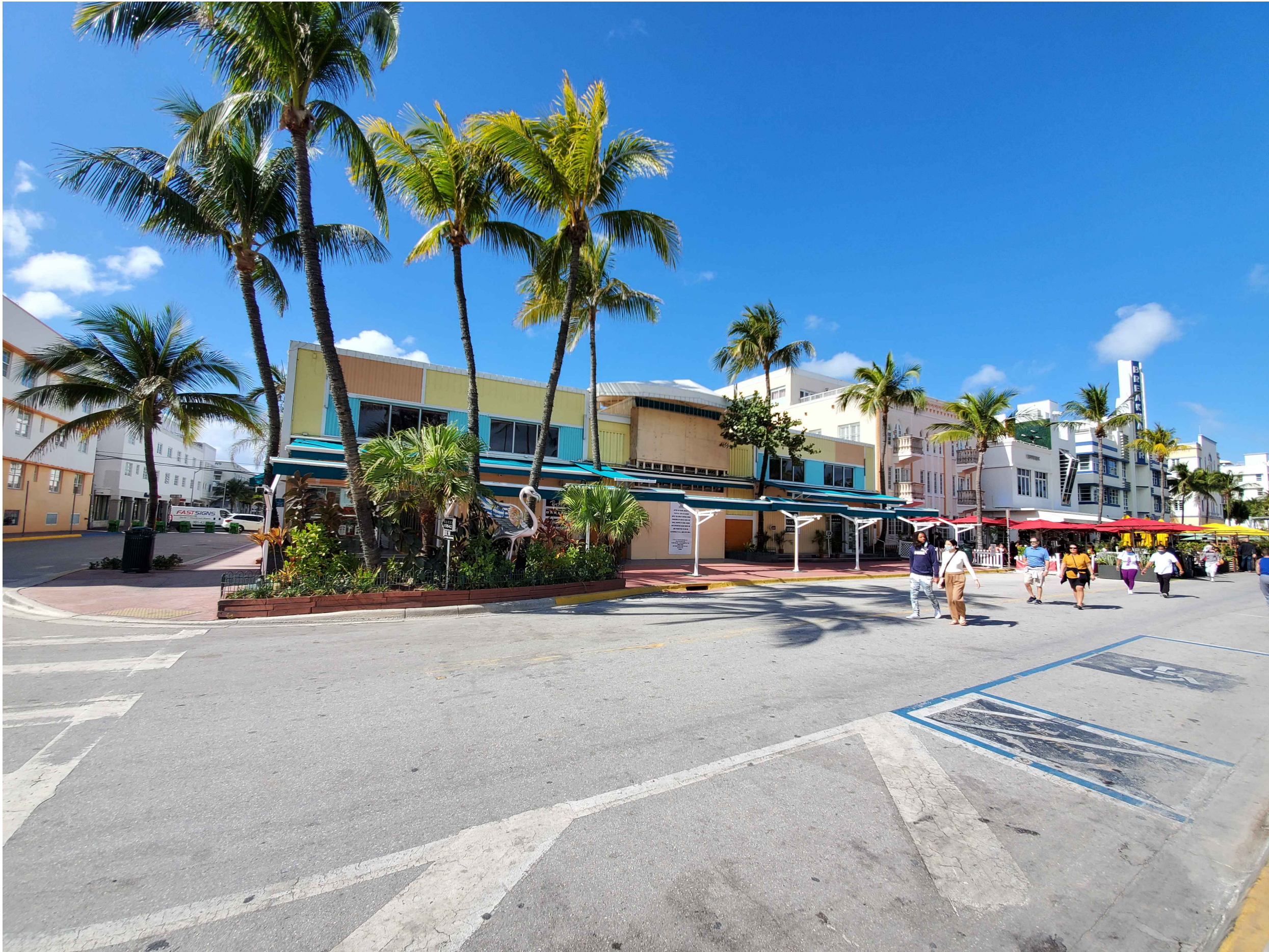
C4 EXTERIOR PICTURE
