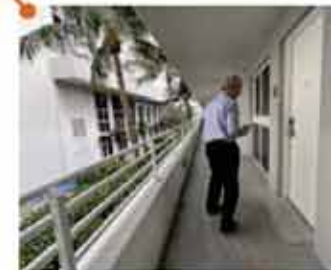
LANAI BUILDING EXTERIOR CORRIDOR
