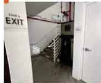
LANAI BUILDING EXTERIOR STAIRS
