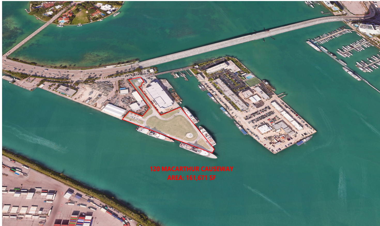
VIEW TOWARD NORTH
