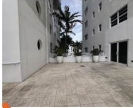
FLEX AREA OUTSIDE OF MEETING ROOMS
