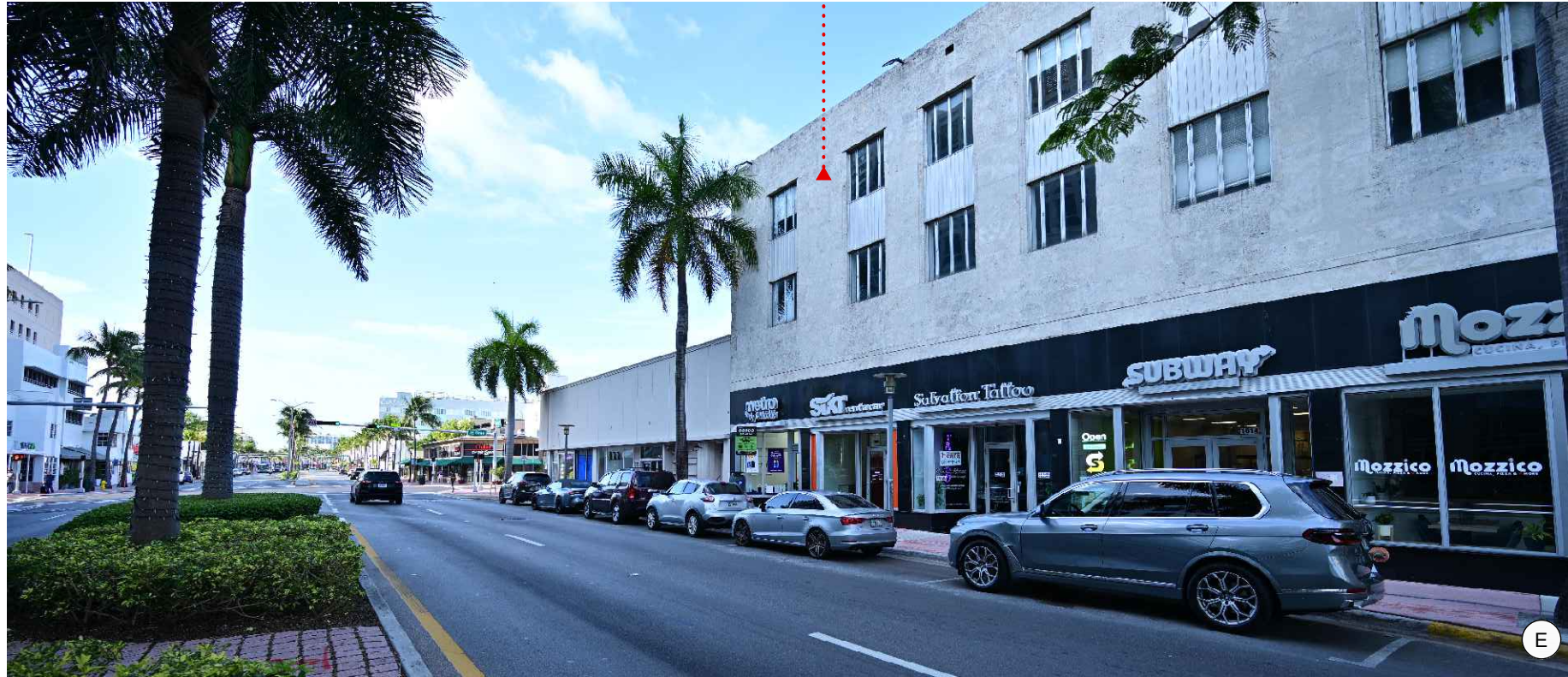
420 LINCOLN RD. EXISTING MULTISTORY BUILDING (NOT IN THE SCOPE OF WORK)
