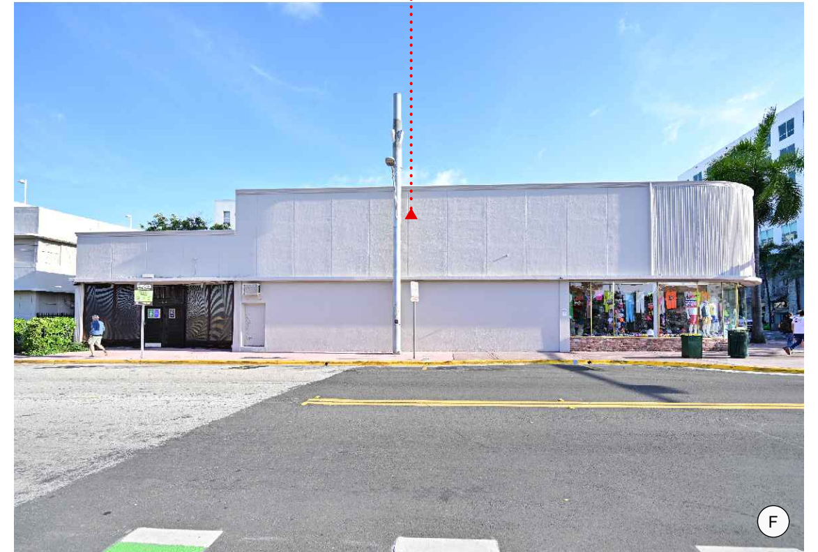
1600 WASHINGTON AVE EXISTING BUILDING TO BE DEMOLISHED SOUTH FACADE
