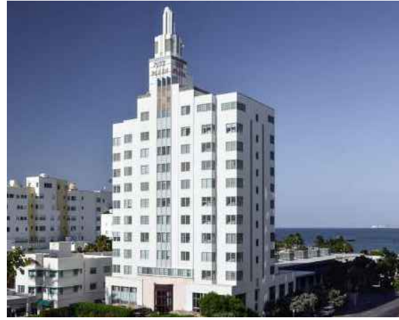
1701 COLLINS AVENUE SLS SOUTH BEACH HOTEL EXISTING THIRTEEN STORY ART-DECO BUILDING
