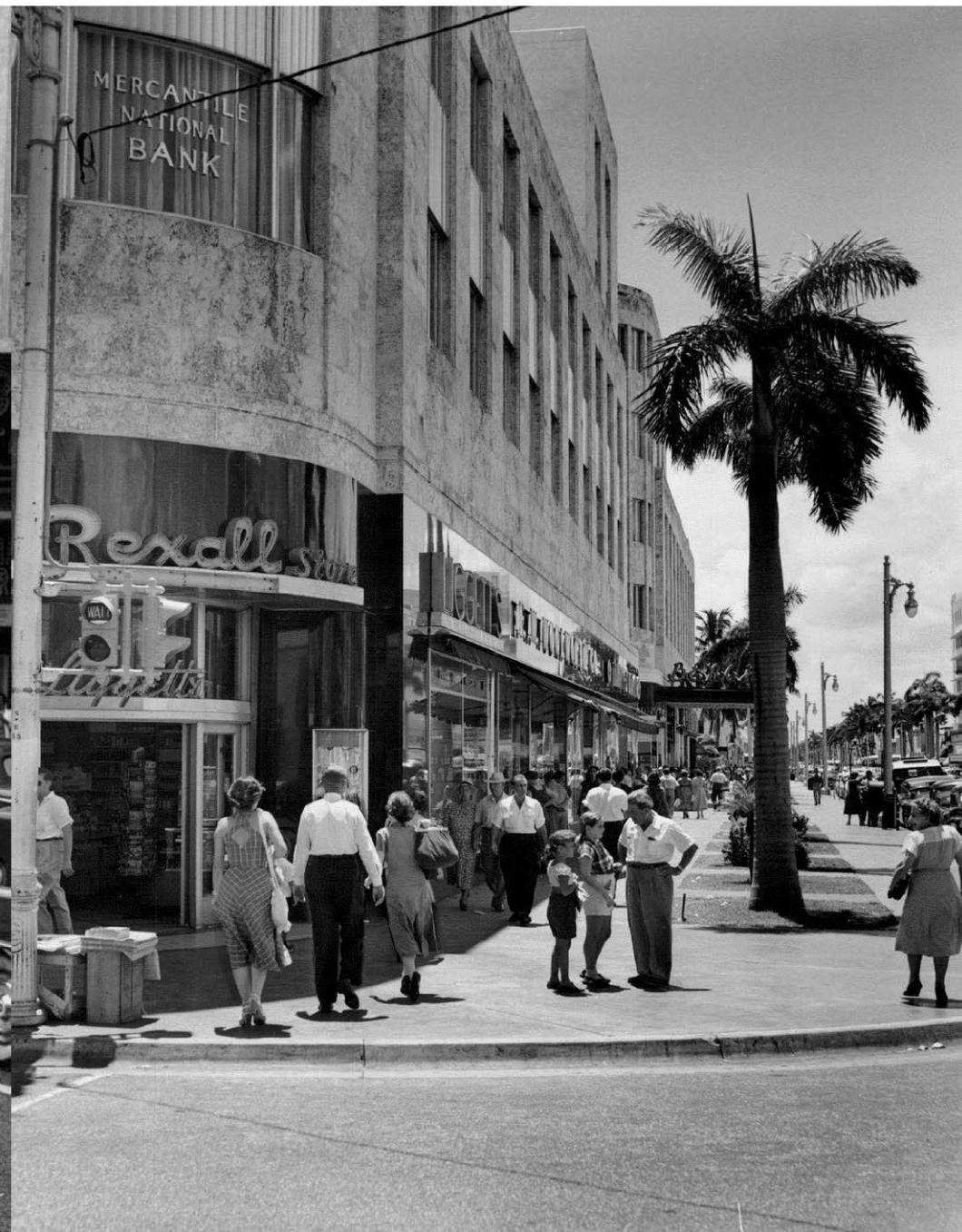
Mercantile National Bank Building (a.k.a. 420 Lincoln Rd. Building) Lincoln Road Mall corner of Washington & Lincoln
