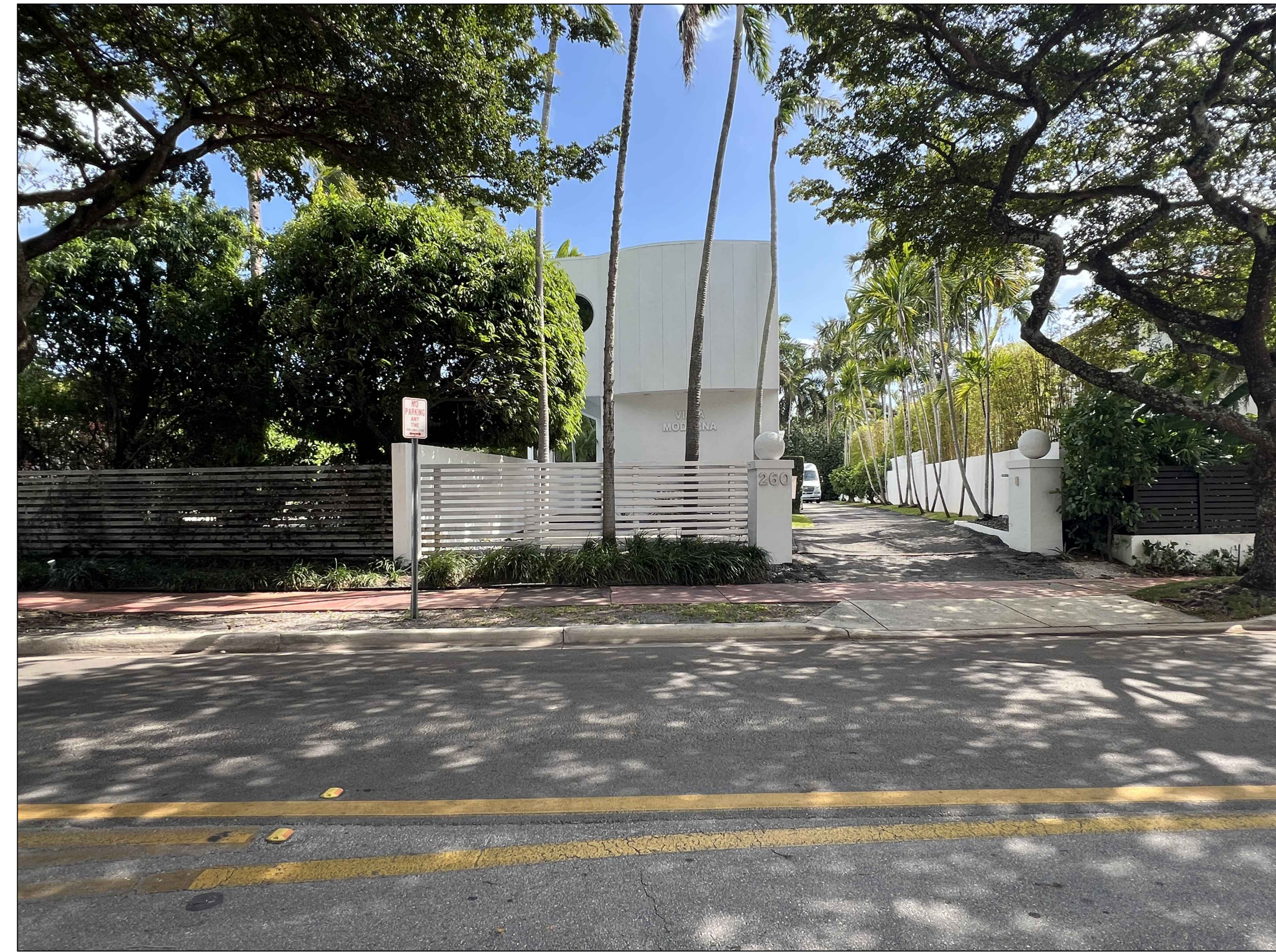
6 260 WEST 35th STREET NORTH FACING
