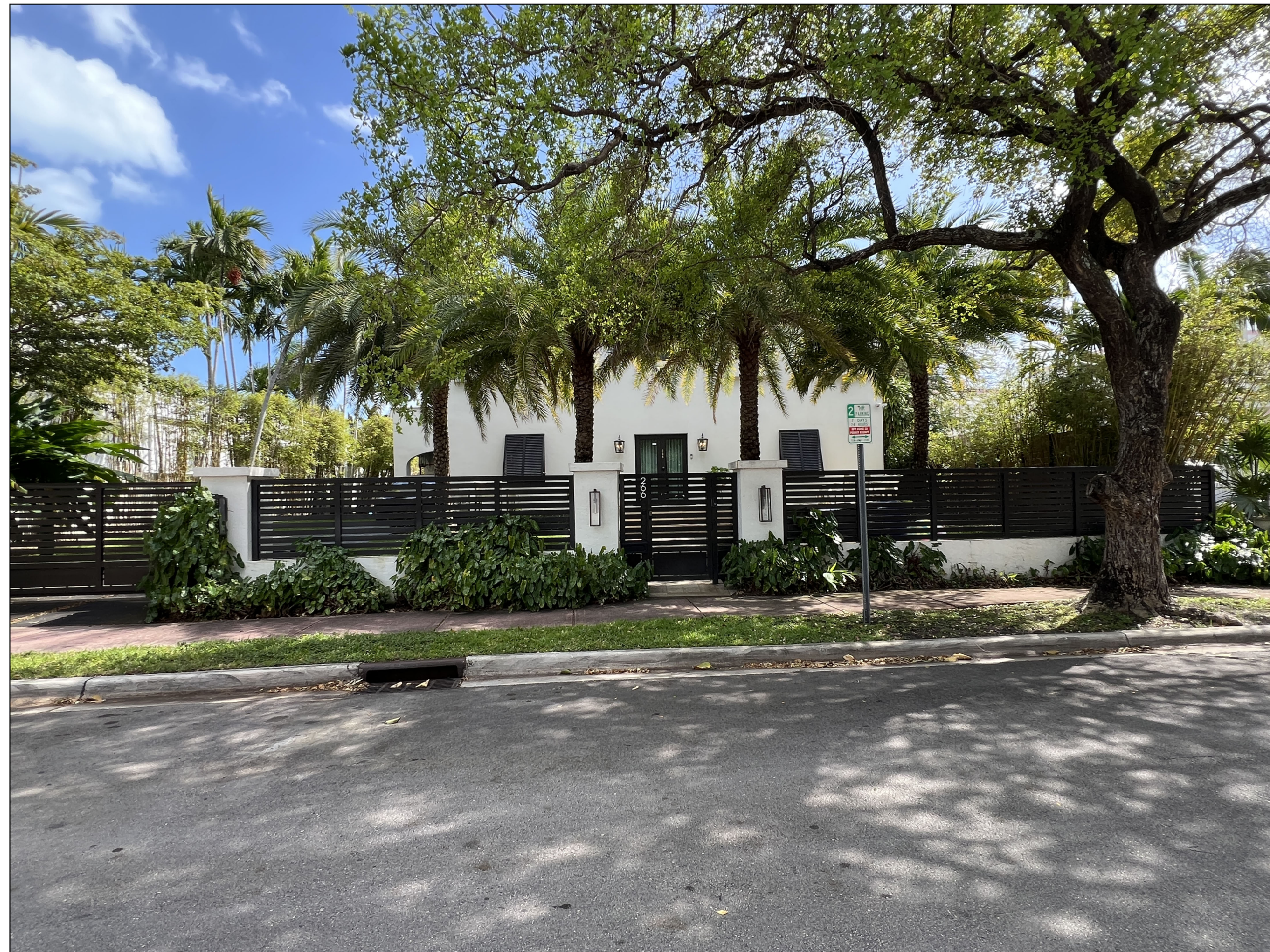
7 266 WEST 35th STREET NORTH FACING
