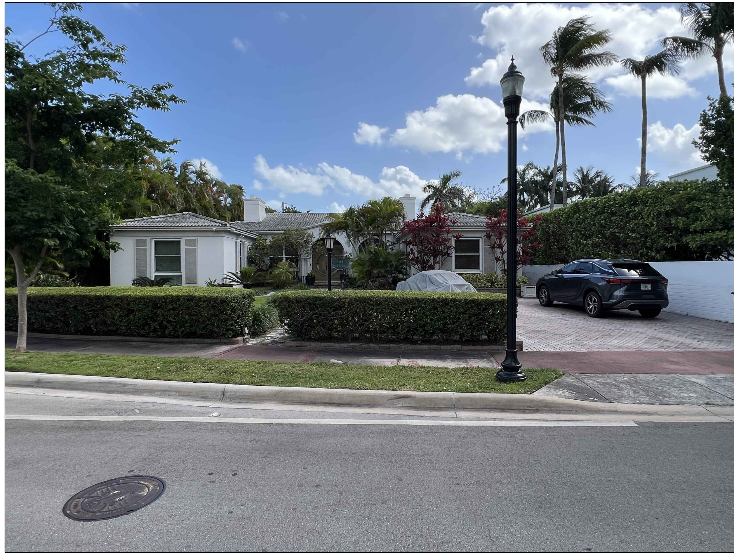
5 254 WEST 35th STREET NORTH FACING
