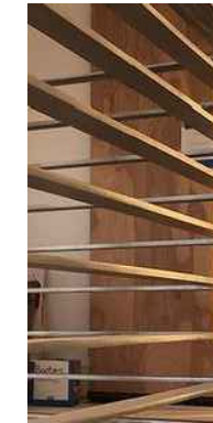
HORIZONTAL RECTANGULAR/FLAT BAR PROFILE GUARD/HANDRAIL (ALL WELDED, NO MECHANICAL CONNECTIONS)
