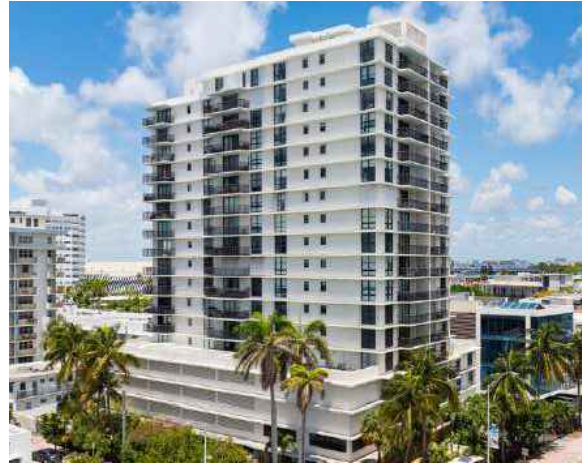
1800 COLLINS AVENUE TOWER 1800 EXISTING NINETEEN STORY BUILDING
