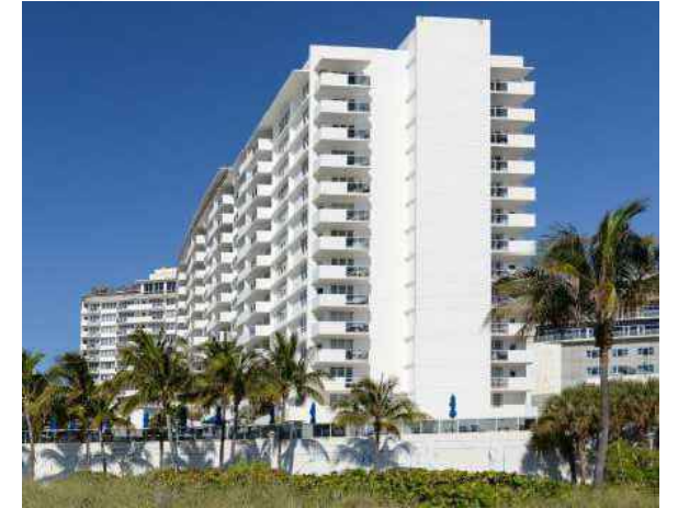
100 LINCOLN RD. DECOPLAGE PROPERTIES EXISTING SIXTEEN STORY BUILDING
