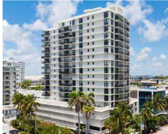
1800 COLLINS AVENUE TOWER 1800 EXISTING NINETEEN STORY BUILDING
