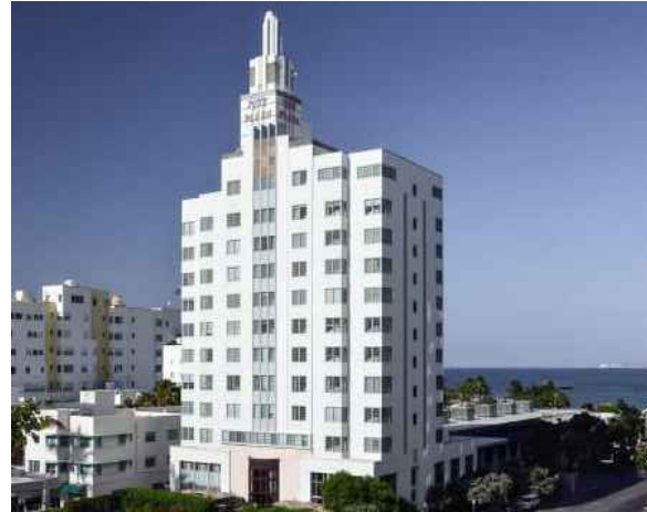
1701 COLLINS AVENUE SLS SOUTH BEACH HOTEL EXISTING THIRTEEN STORY ART-DECO BUILDING
