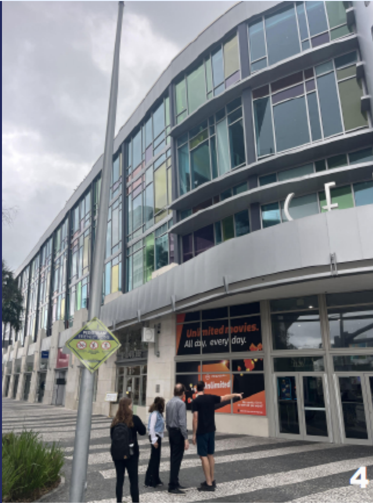
NORTH ELEVATION, FRONTING LINCOLN ROAD, LOOKING AT ENTRANCE OF BUILDING
