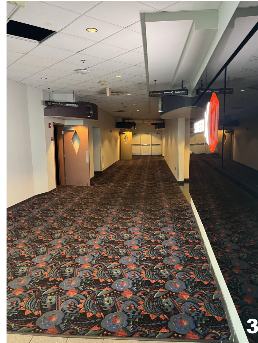
SECOND LEVEL THEATER HALLWAY
