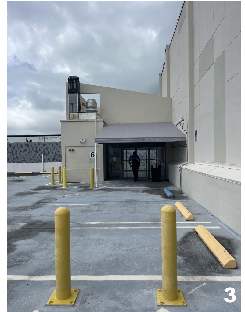
THIRD FLOOR EXTERIOR PARKING LOOKING WEST
