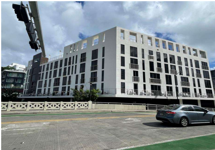
12 WEST AVENUE BRIDGE / ADJACENT HOTEL
