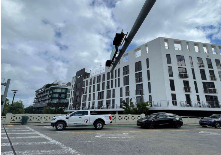
13 WEST AVENUE BRIDGE / ADJACENT HOTEL
