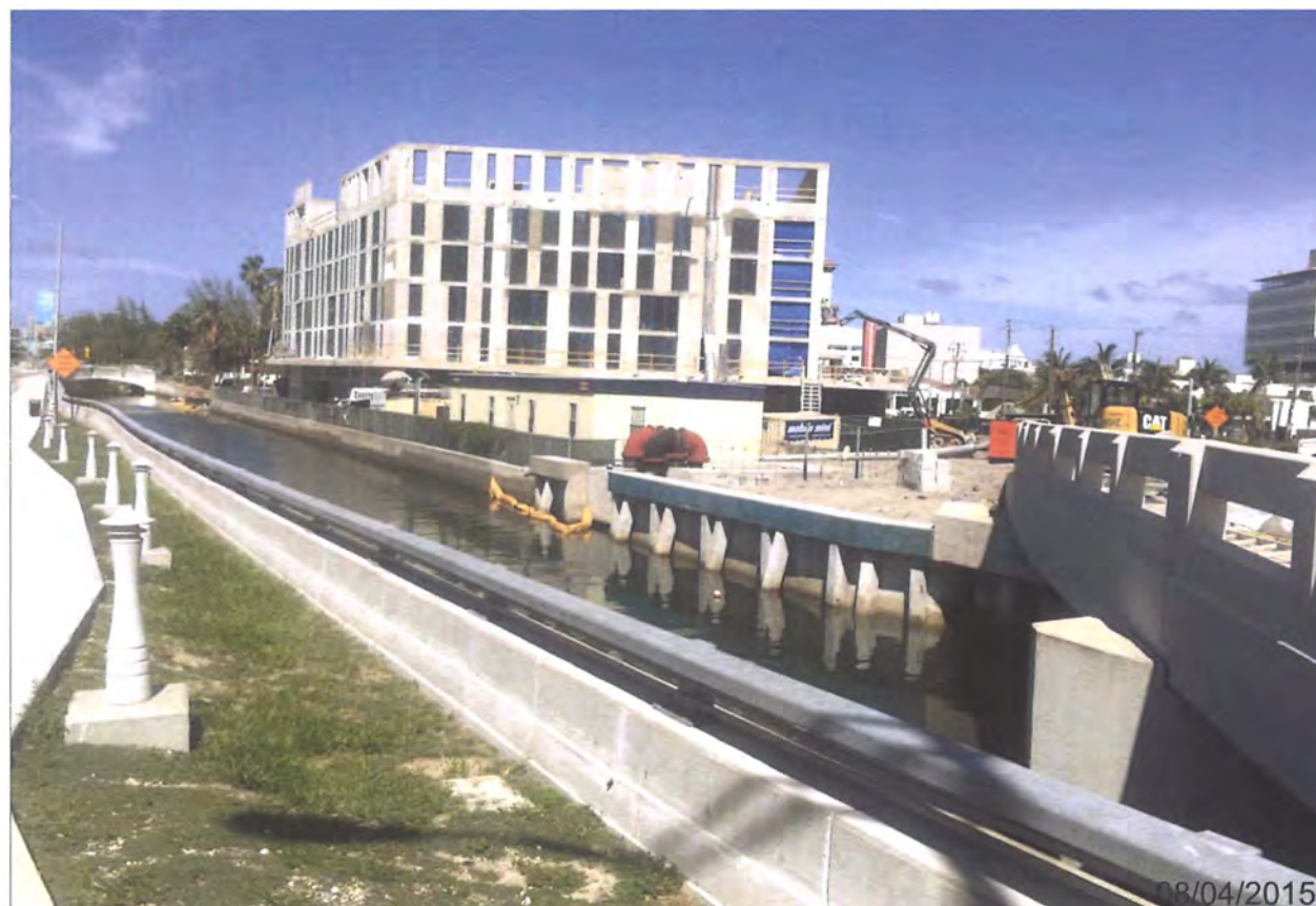
12 WEST AVENUE BRIDGE / ADJACENT SITE
