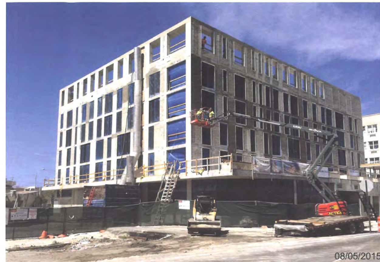
11 ADJACENT PROPERTY 5 STORY HOTEL
