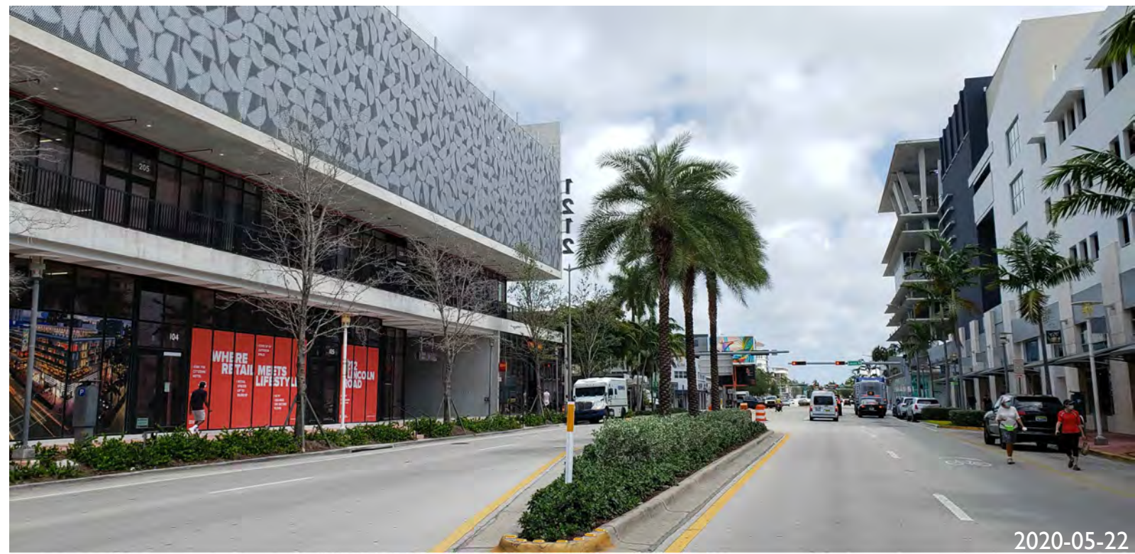
8. 1212 LINCOLN ROAD BUILDING - EAST FACADE
