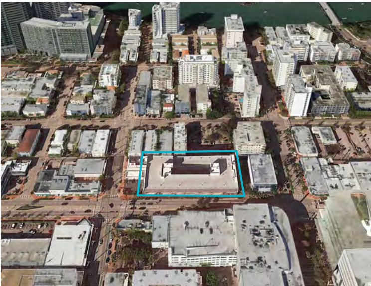
SITE AERIAL - EAST
