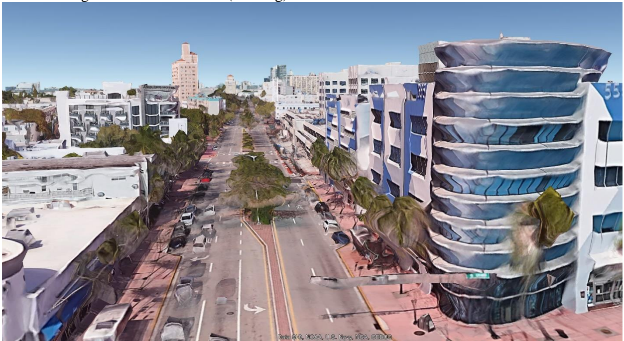
View looking north from 5 th Street (existing):
