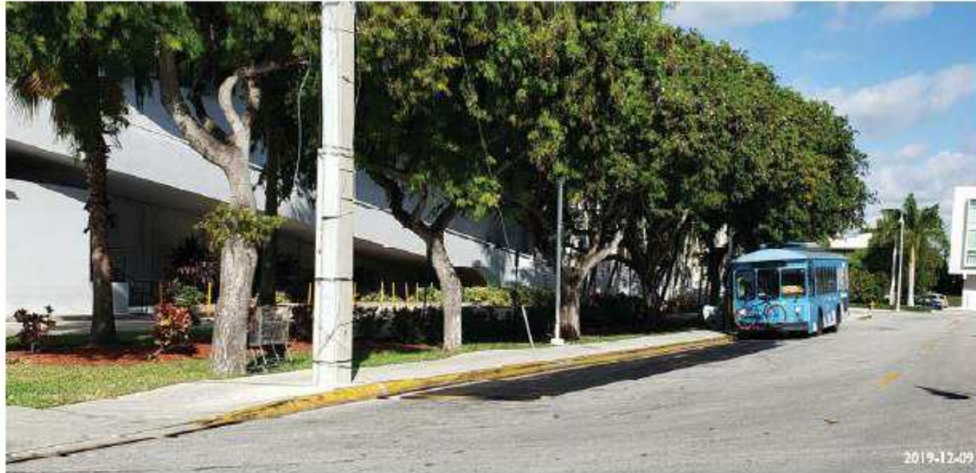
16. VIEW OF PUBLIX GARAGE ON WEST AVENUE AND 20TH STREET
