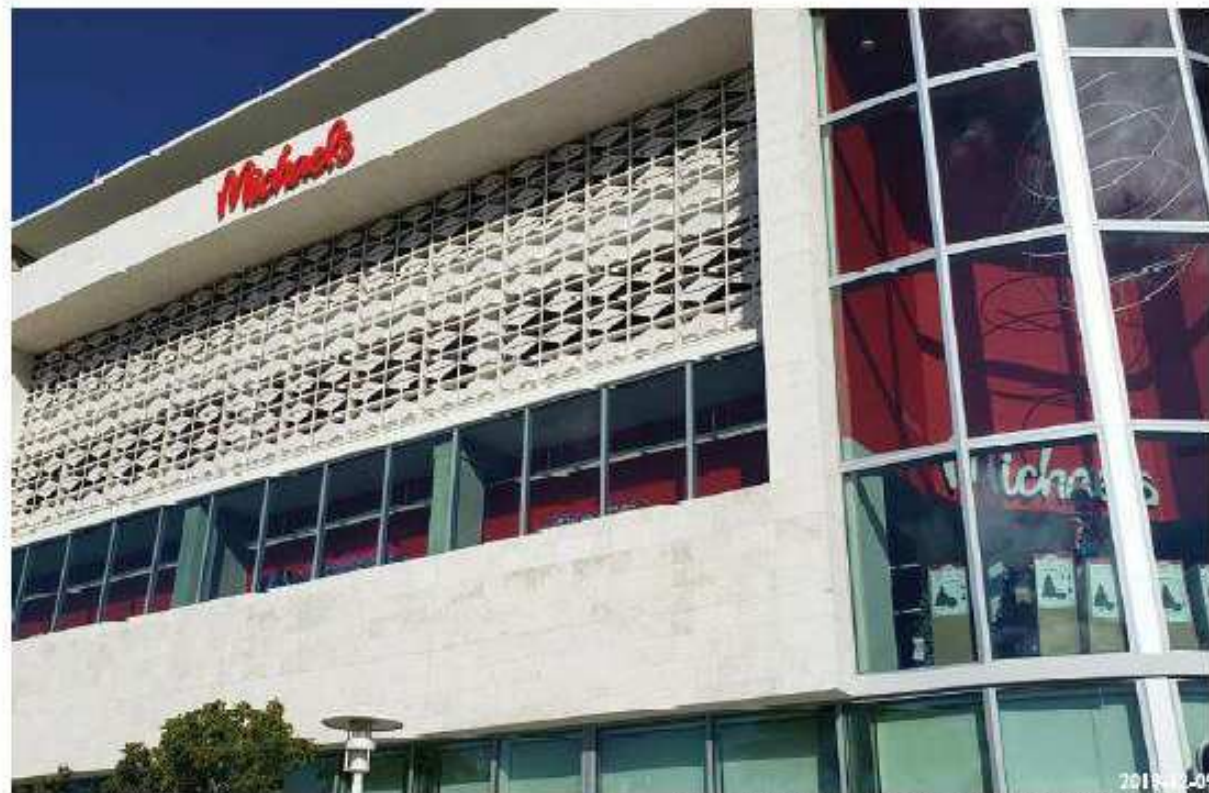
6. VIEW OF FACADE DETAIL AT NEIGHBORING BUILDING
