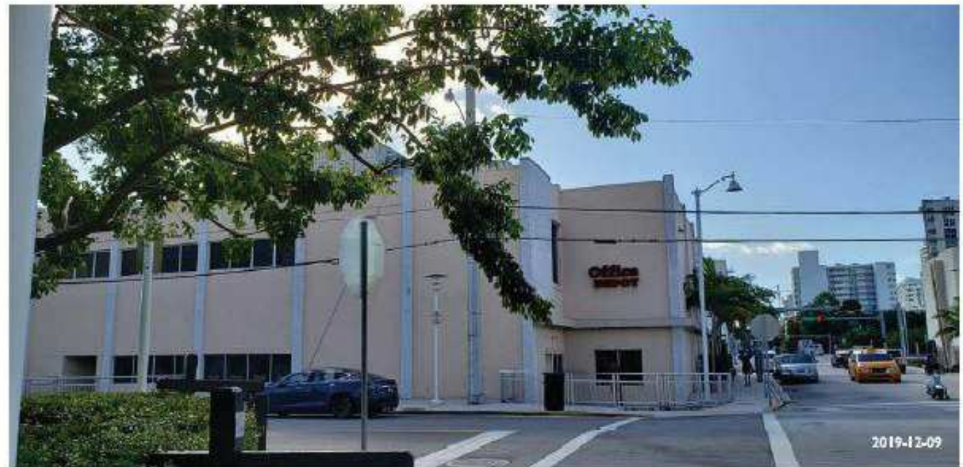
15. VIEW OF OFFICE DEPOT STORE FACING SOUTH-EAST
