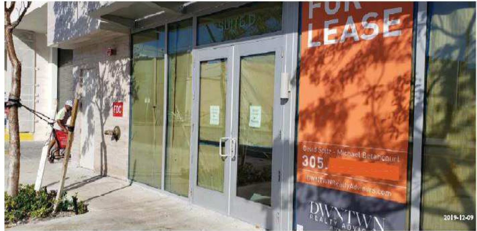
9. VIEW OF NEIGHBORING BUILDING AT RETAIL AREA AT 18TH STREET
