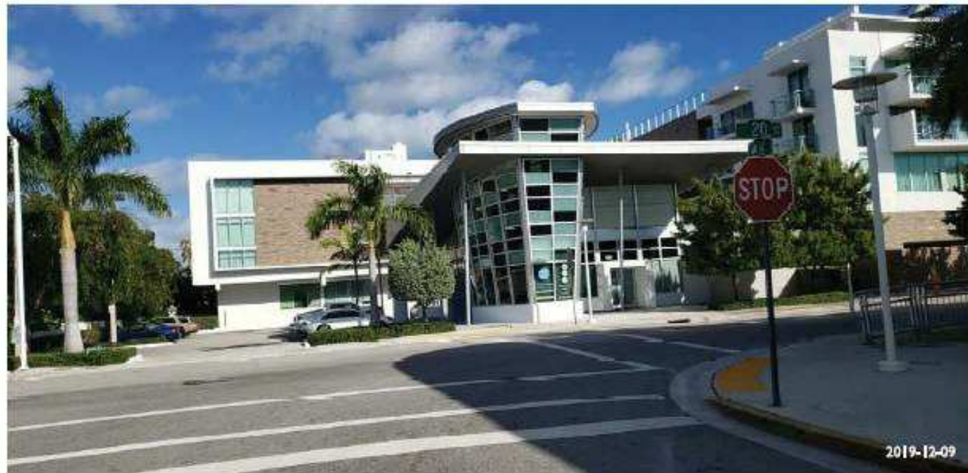
18. VIEW OF OFFICE BUILDING ON WEST AVENUE AND 20TH STREET
