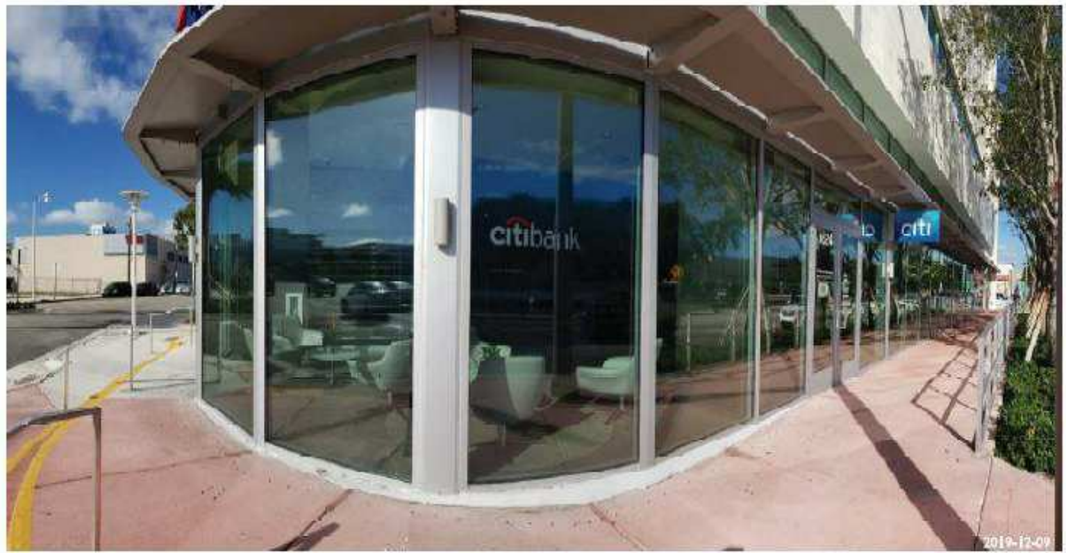
2019-12-09 5. VIEW OF NEIGHBORING BUILDING AT RETAIL AREA FACING ALTON ROAD AND 18TH STREET
