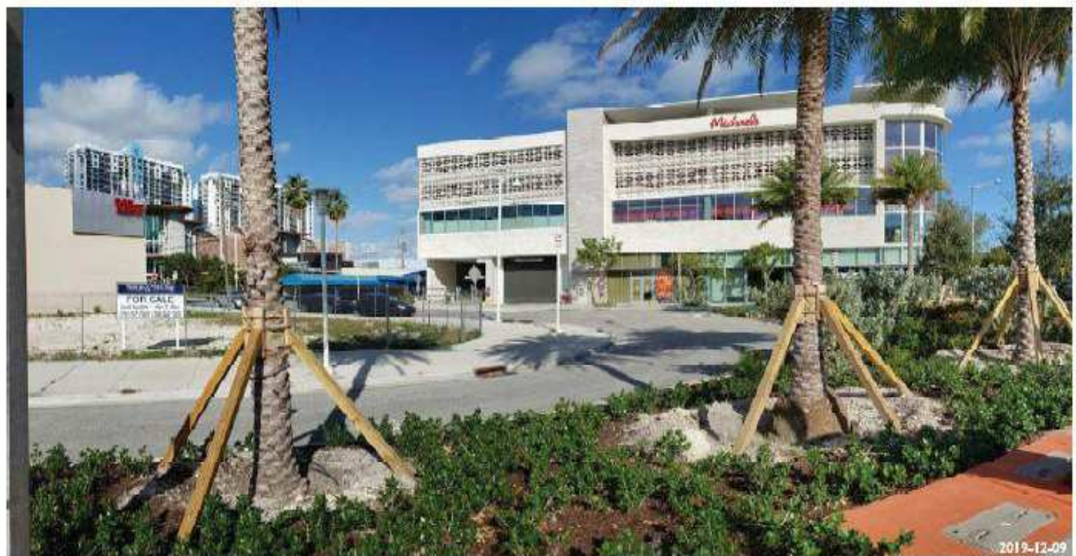
2019-12-09 7. VIEW OF SITE FACING NORTH-WEST
