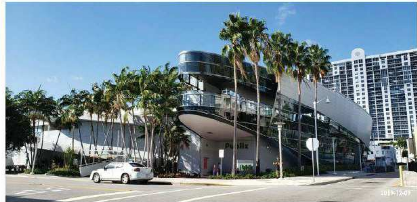
19. VIEW OF PUBLIX ON WEST AVENUE AND 20TH STREET
