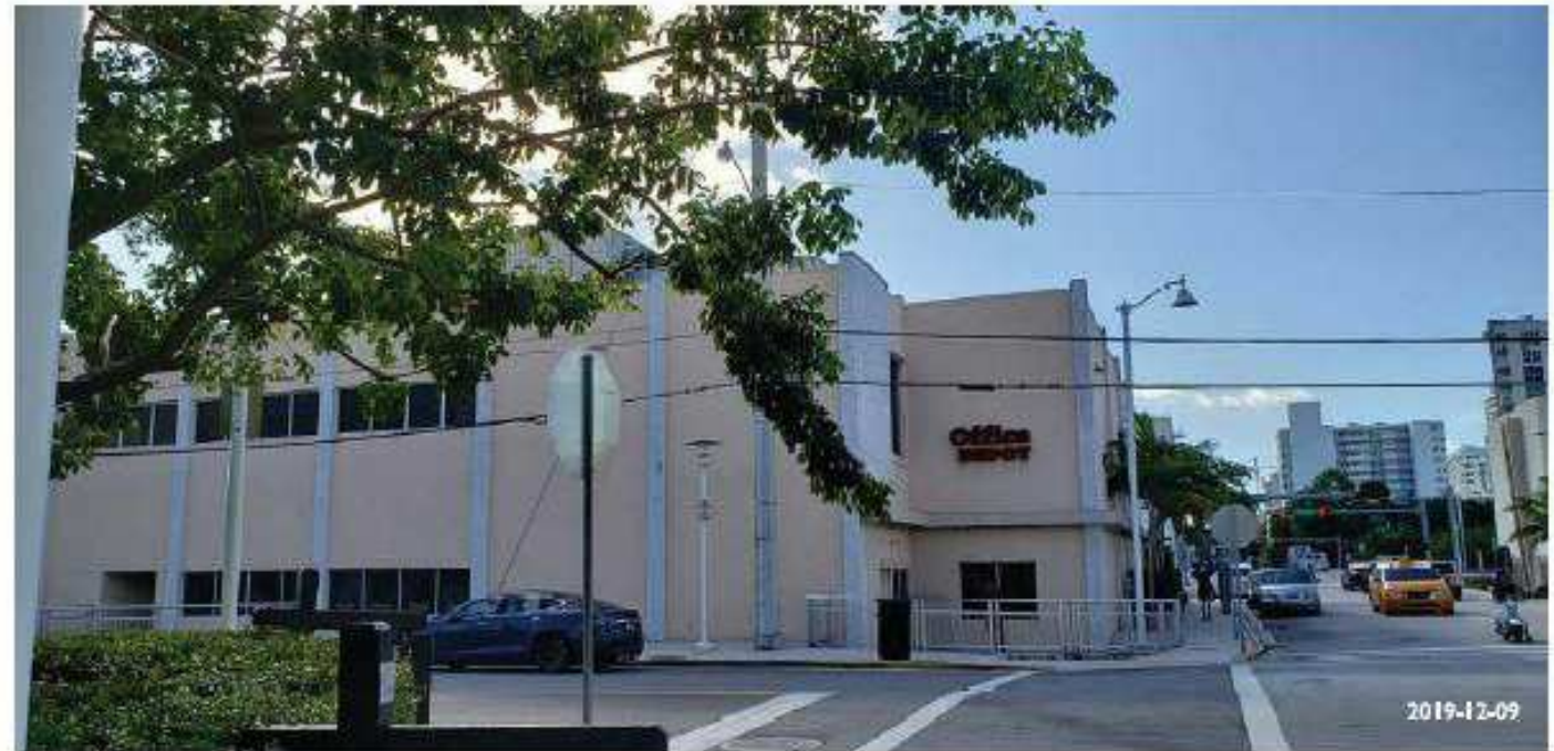
15. VIEW OF OFFICE DEPOT STORE FACING SOUTH-EAST
