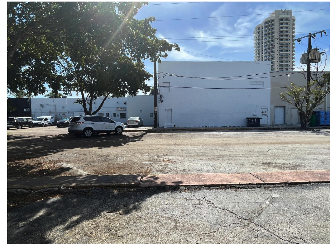
5. CVS and Surf Buildings facing the Collins Ct
