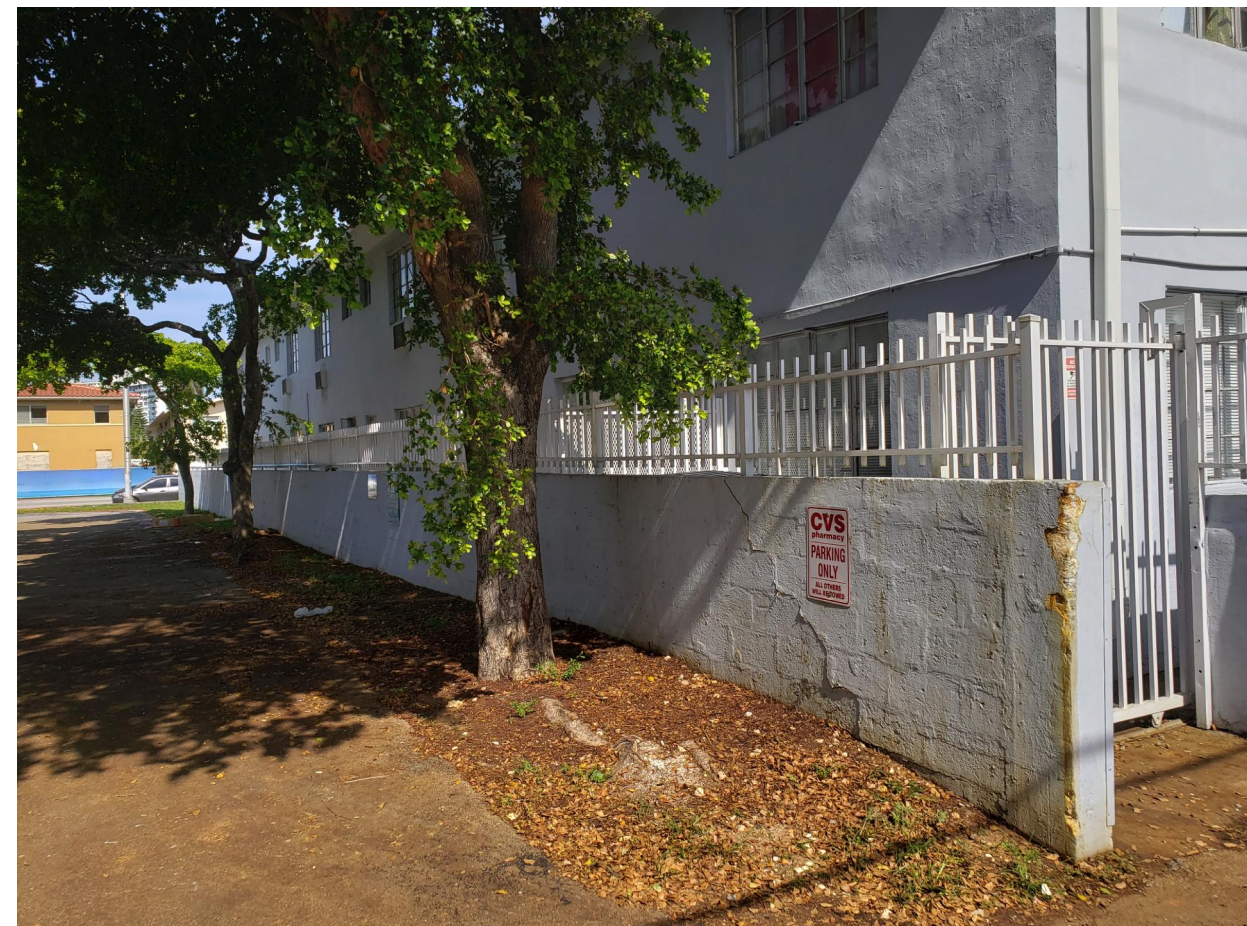
8. Adjacent Neighboring Building
