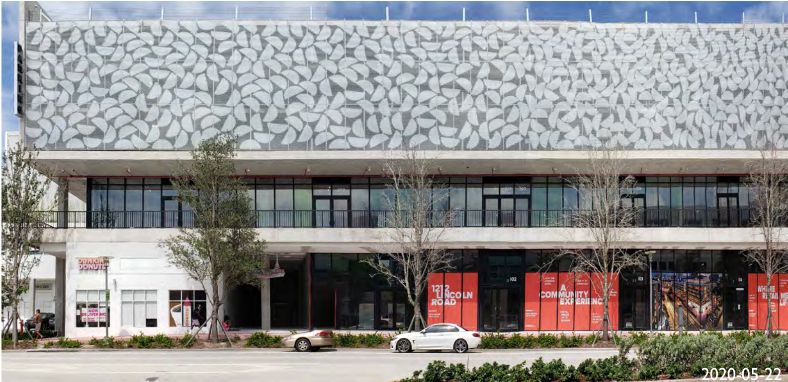
1. 1212 LINCOLN ROAD BUILDING - SOUTHEAST PORTION
