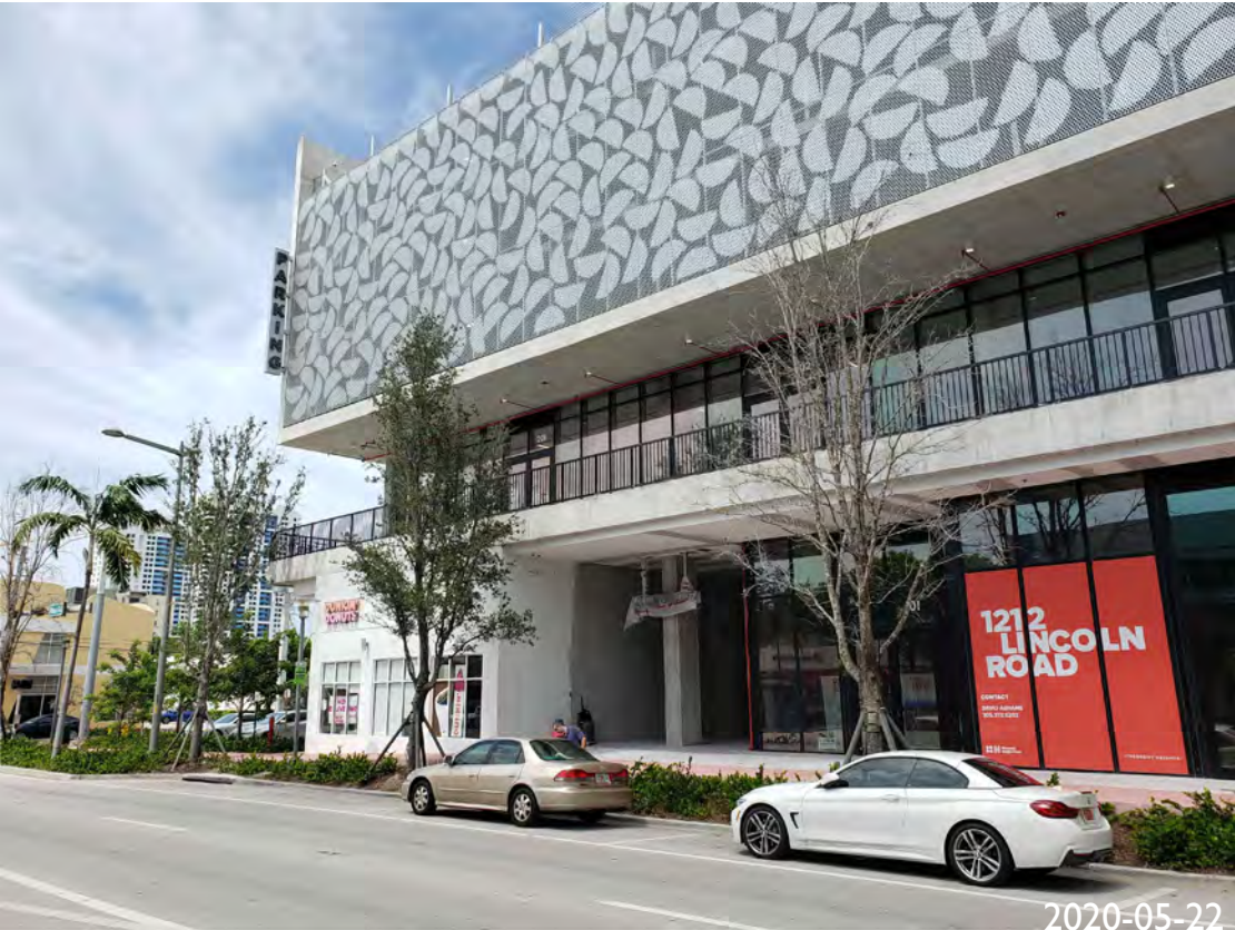
4. 1212 LINCOLN ROAD BUILDING - SOUTHEAST PORTION
