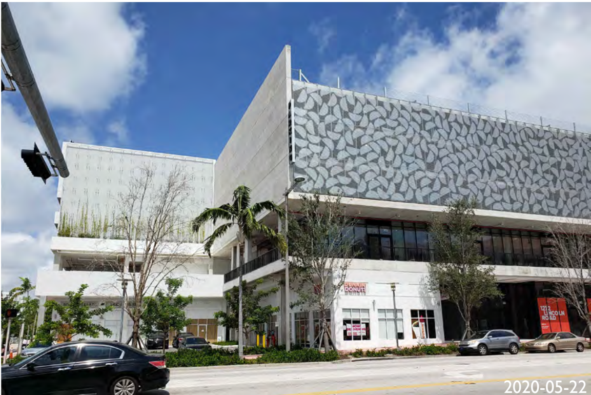
2. 1212 LINCOLN ROAD BUILDING - SOUTHEAST PORTION
