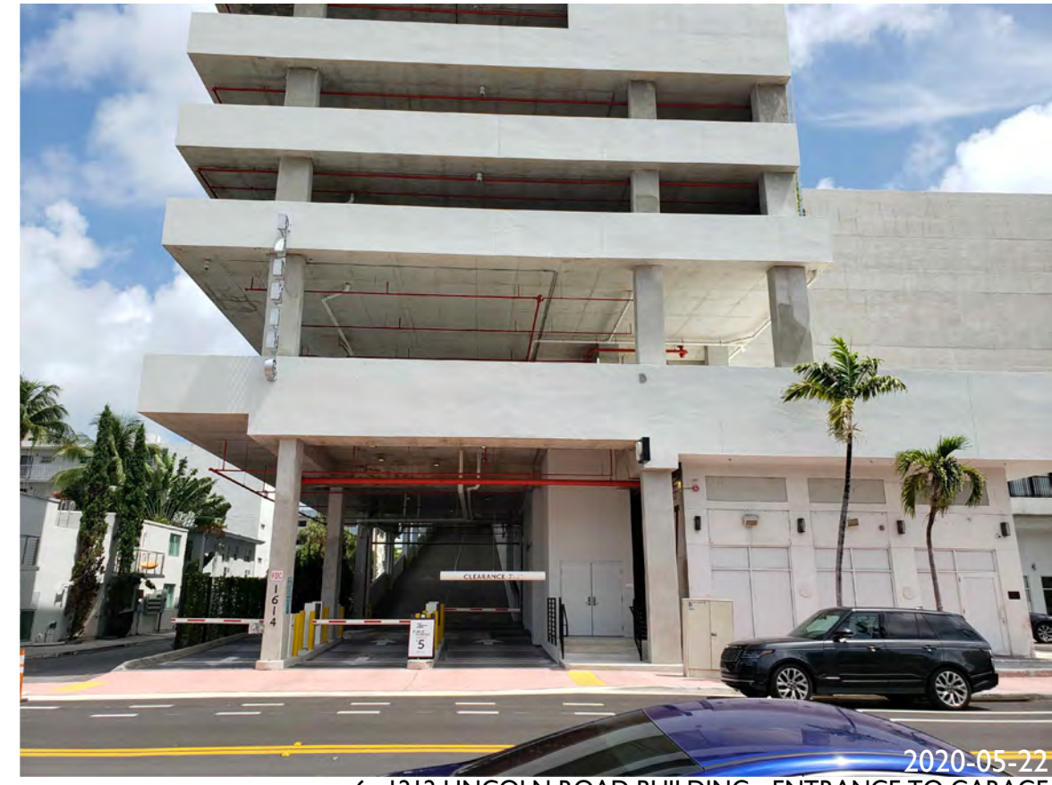
6. 1212 LINCOLN ROAD BUILDING - ENTRANCE TO GARAGE
