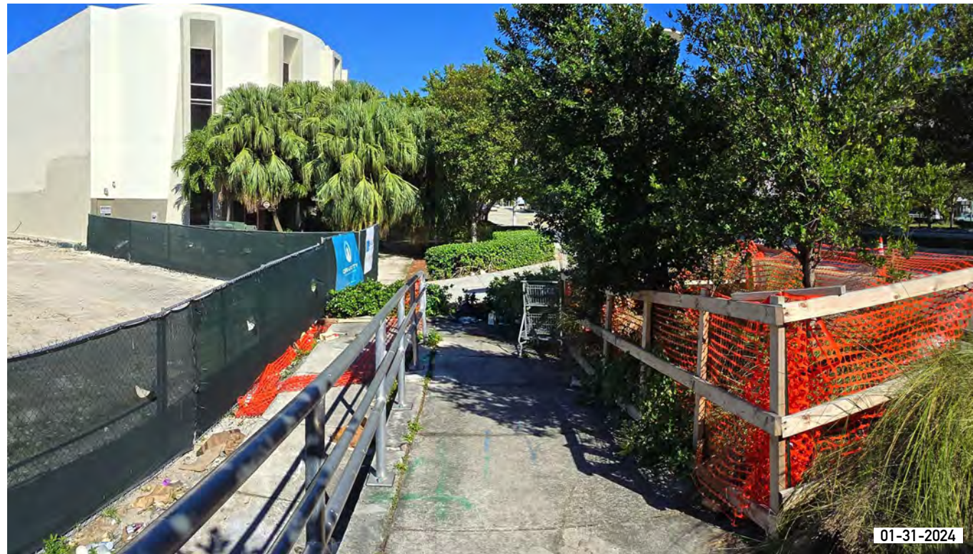
16. ACCESSIBLE RAMP AT FRONT OF LOT
