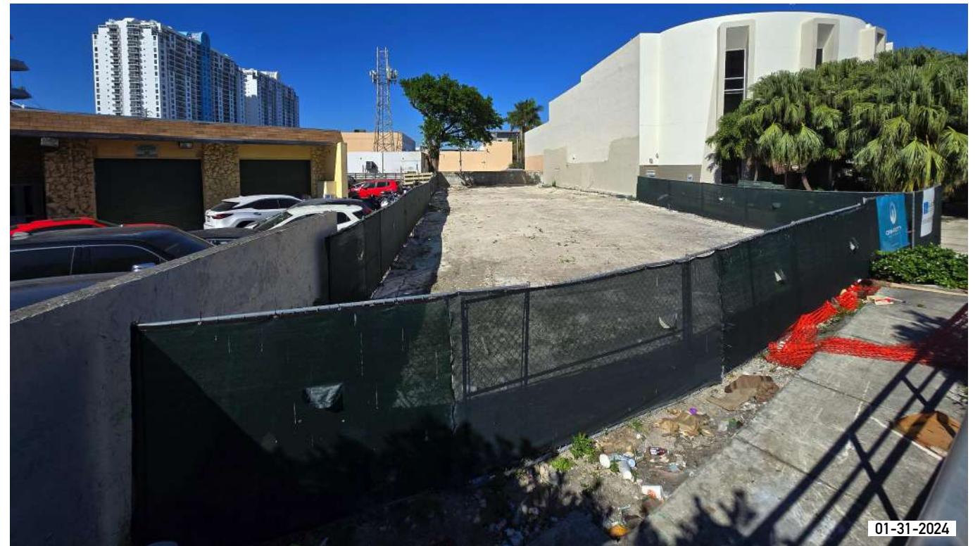
17. FRONT VIEW FROM DADE BOULEVARD
