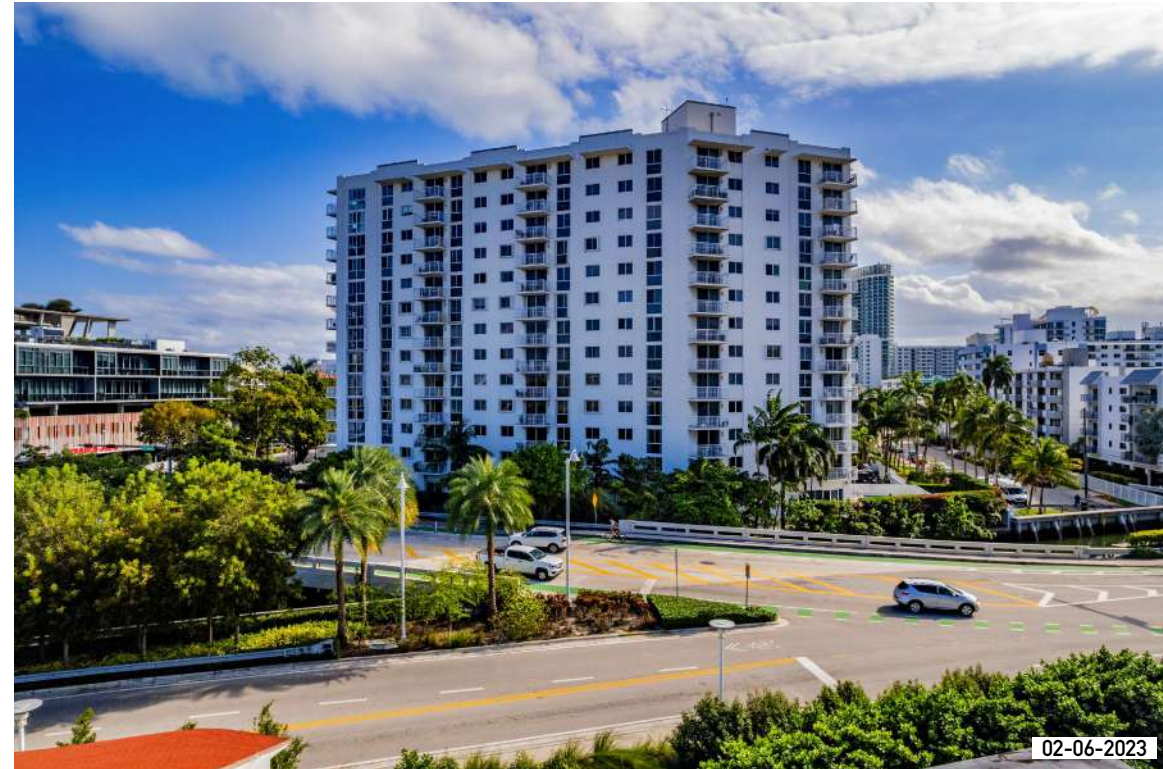
4. VIEW TOWARDS COLLINS CANAL
