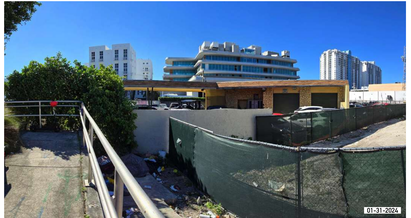
15. SOUTH ENTRANCE AND RAMP
