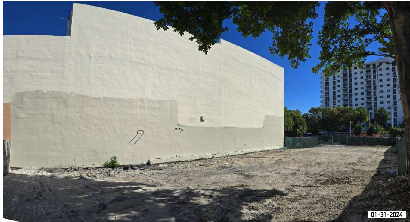
14. SOUTH WEST CORNER OF SITE
