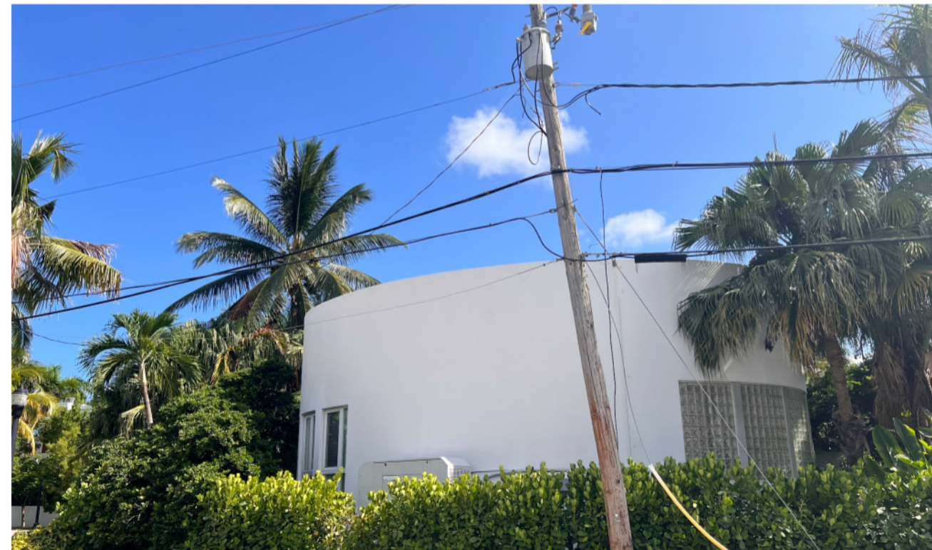
8 312 PALM AVENUE EXISTING TWO-STORY RESIDENCE
