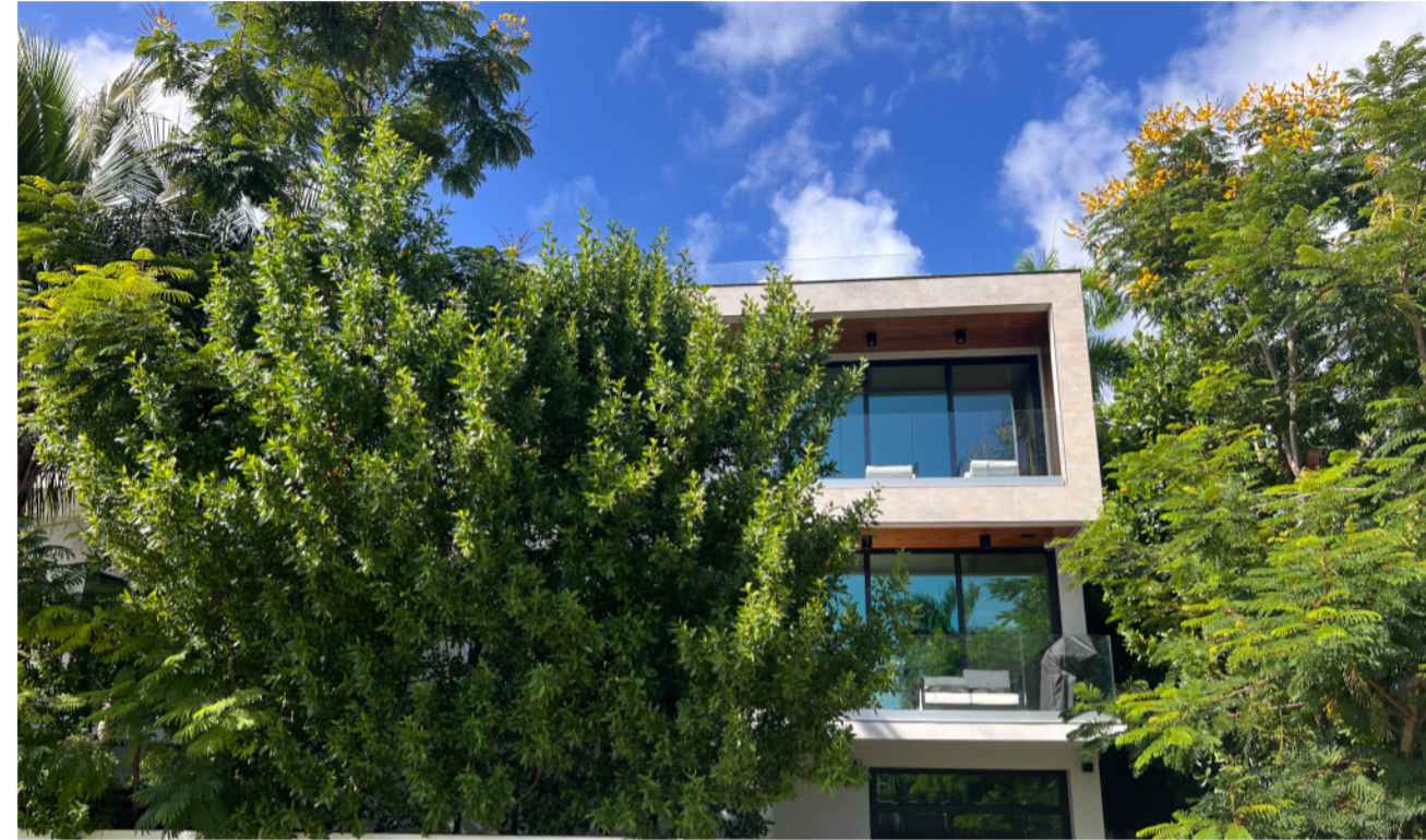
6 288 PALM AVENUE EXISTING TWO-STORY RESIDENCE
