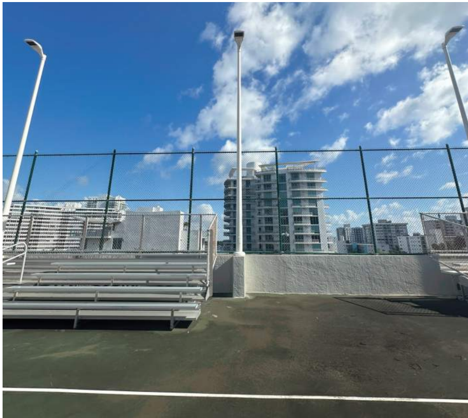
Existing Basketball Court
