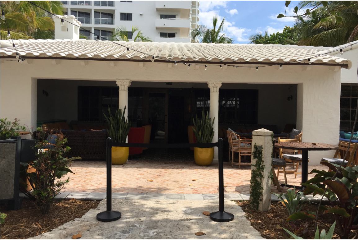
VIEW 5: NOUTH ENTRANCE FROM POOL
