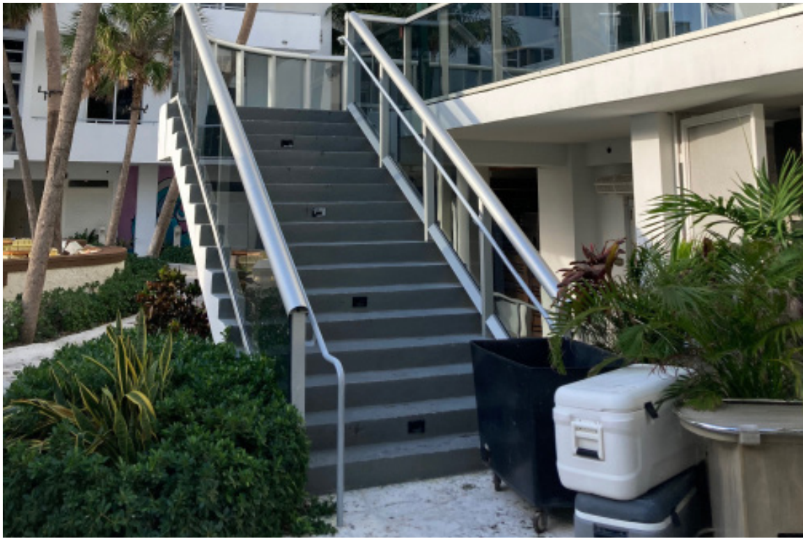
VIEW 2: SECOND FLOOR ACCESS
