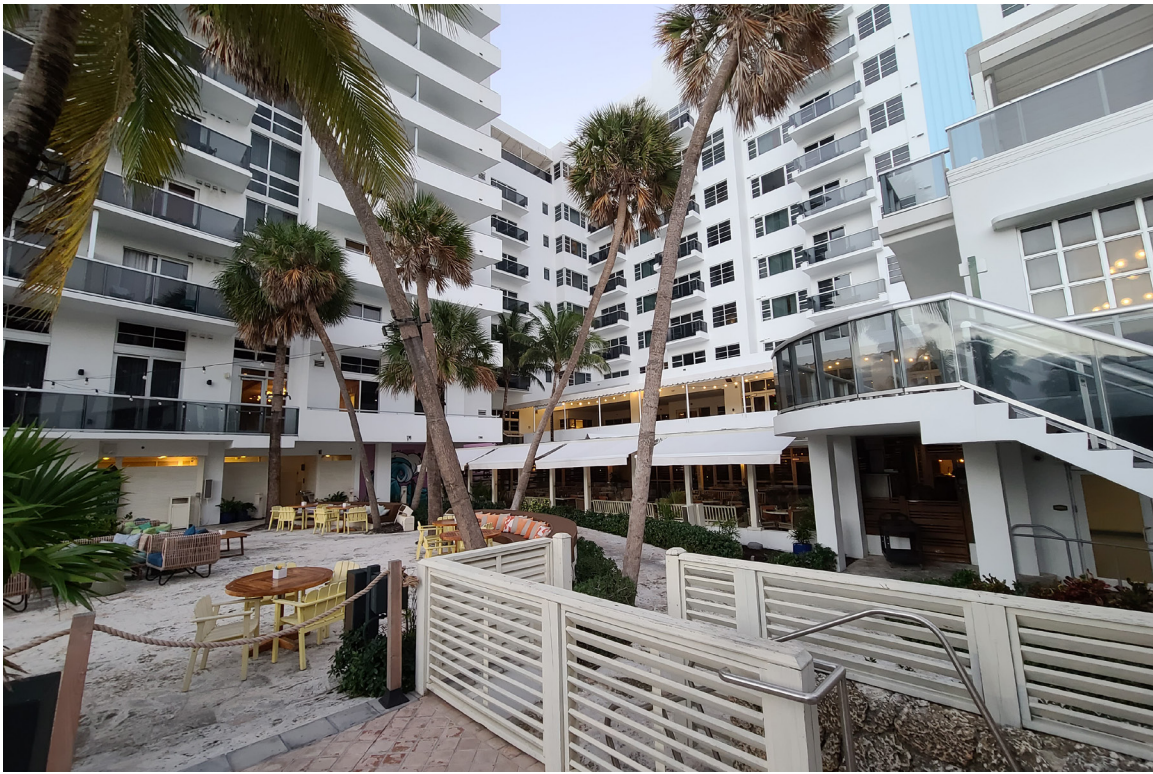
VIEW 1: SECOND FLOOR ACCESS
