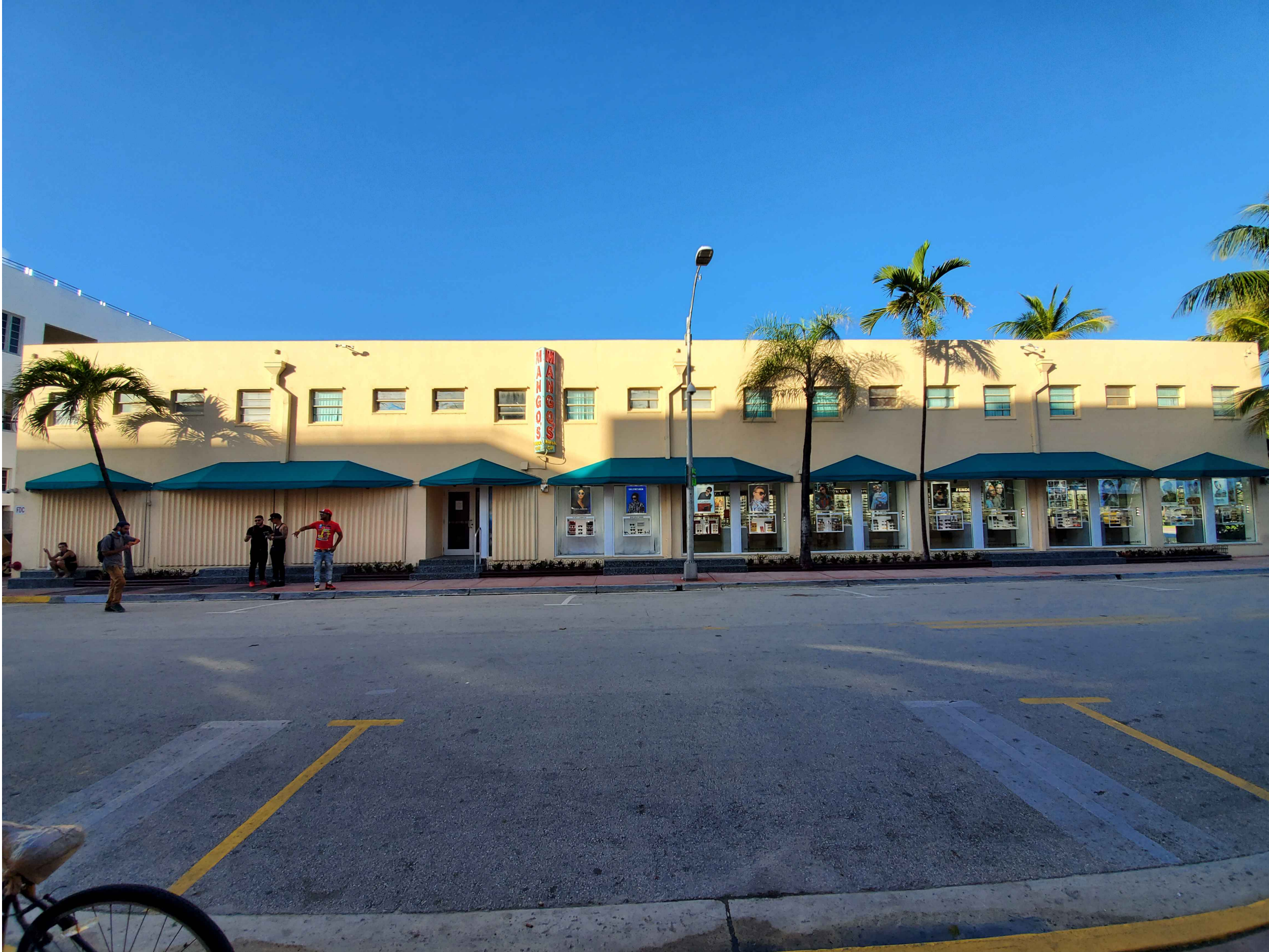
A1 EXTERIOR PICTURE
