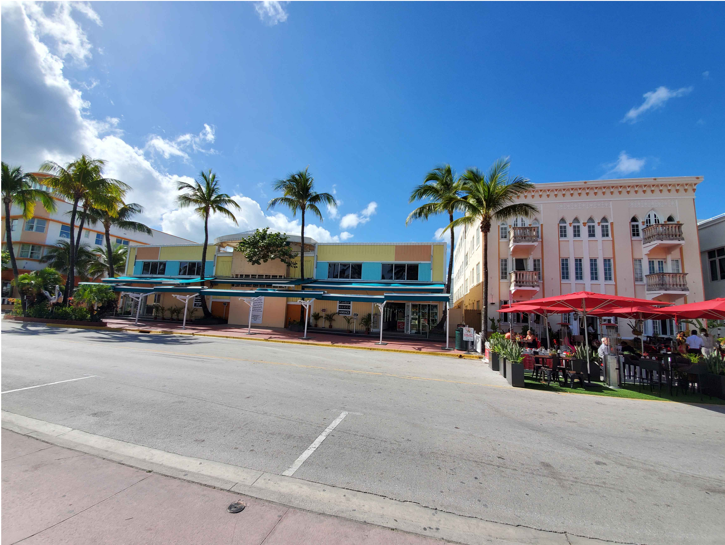
C1 EXTERIOR PICTURE
