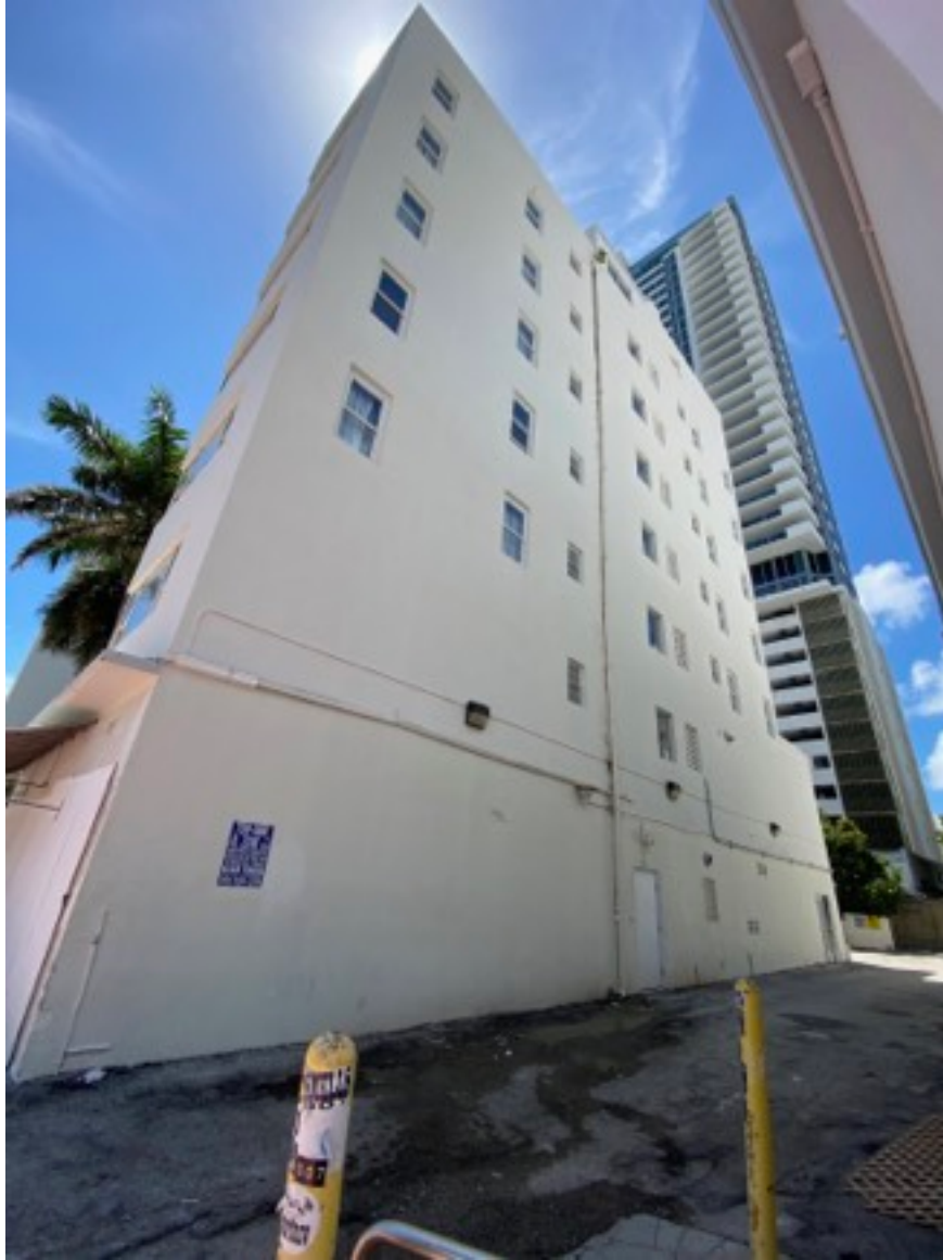
PHOTO LEFT: WEST ELEVATION OF BUILDING AT ALLEY ENTRANCE FROM 21st STREET..
